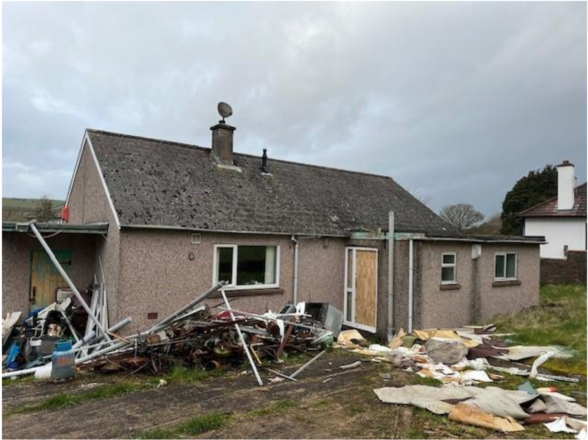
PHOTOGRAPH OF REAR (SOUTHEAST) ELEVATION TAKEN FROM REAR GARDEN.
