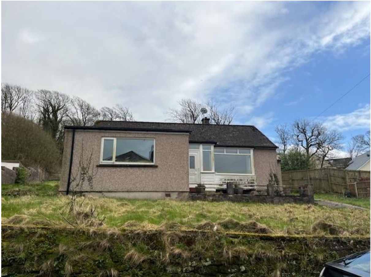
PHOTOGRAPH OF FRONT (NORTHWEST) ELEVATION TAKEN FROM PUBLIC HIGHWAY.
