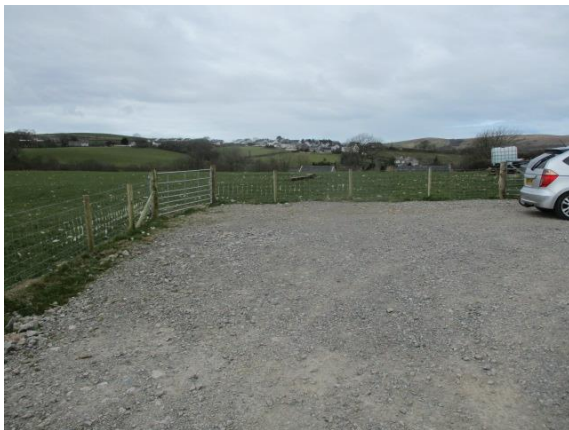
Hardstanding and gate
