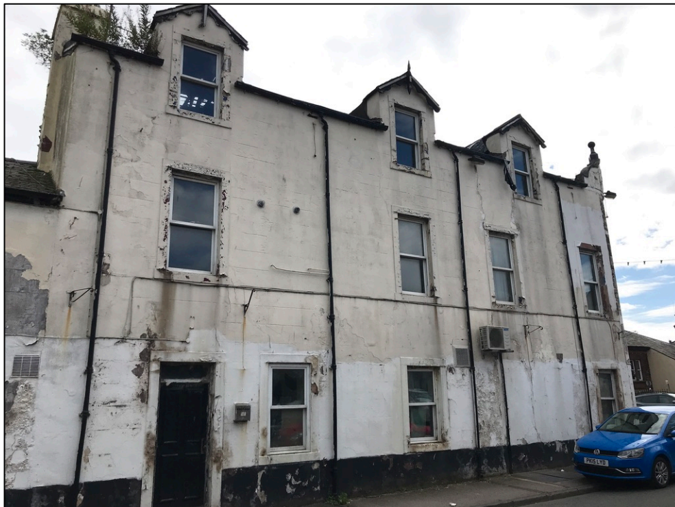
2. West elevation facing North Street.
