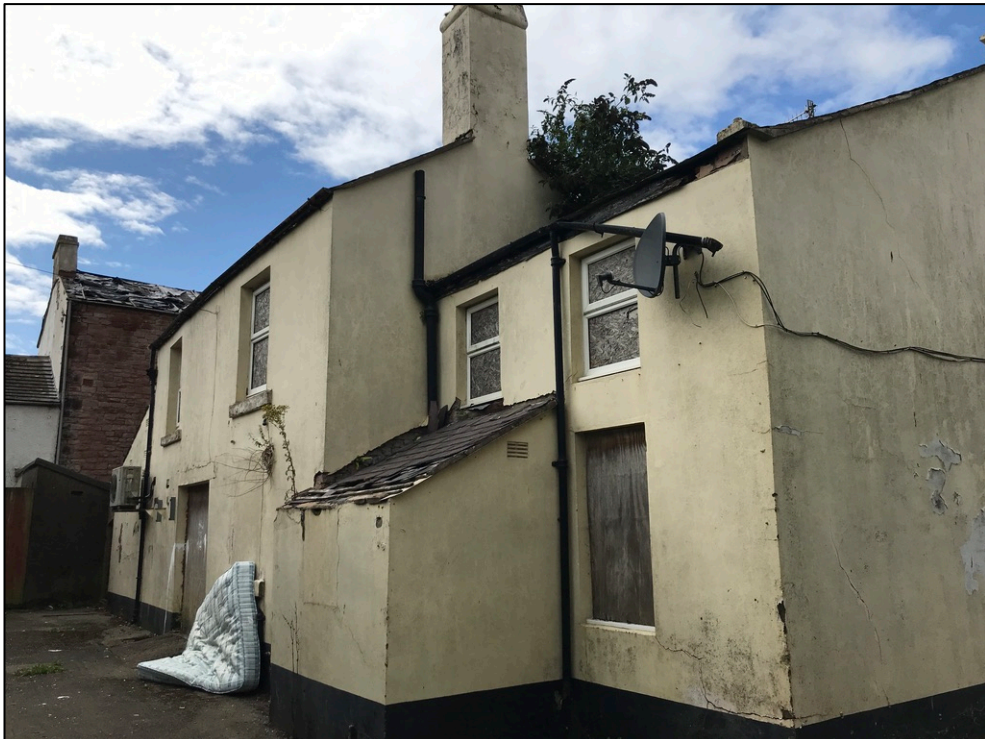
4. East elevation of rear wing (formerly The Albert Public House) facing the rear courtyard.
