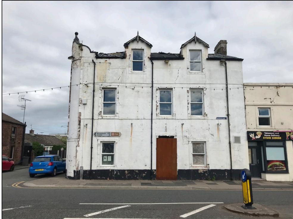
1. South elevation facing High Street.
