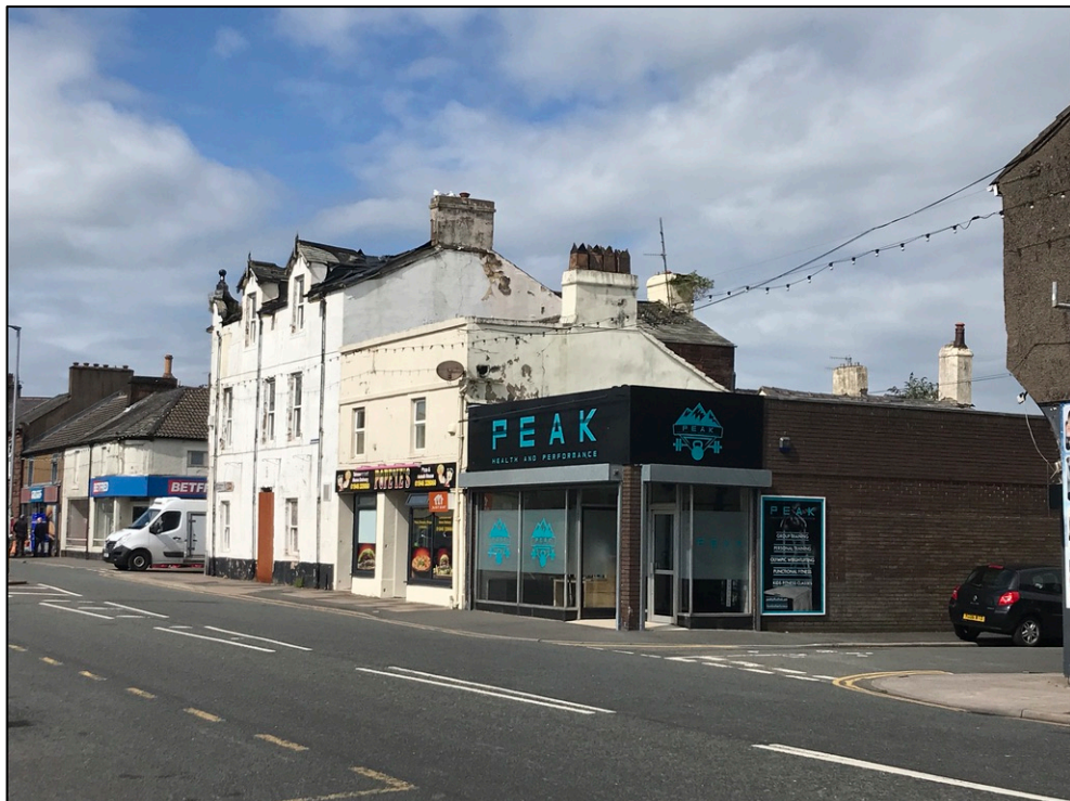
6. Oblique view of the site from the west, in context with neighbouring properties on High Street.
