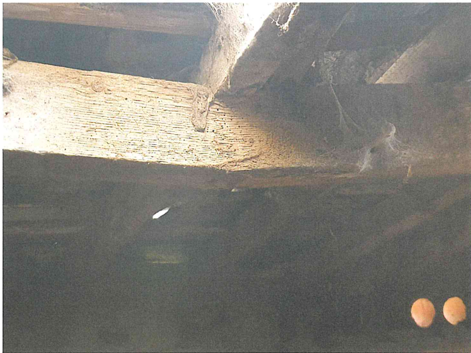
PHOTOGRAPH 04 FAILED ROOF PURLIN
