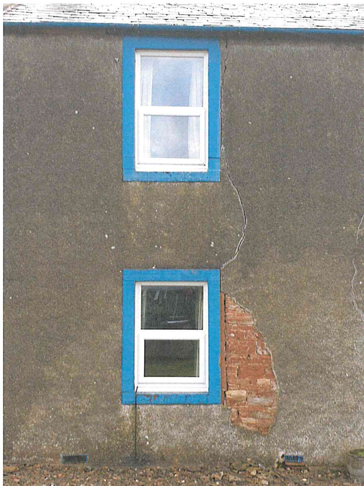
PHOTOGRAPH 02 VIEW ON CRACK TO FRONT ELEVATION
