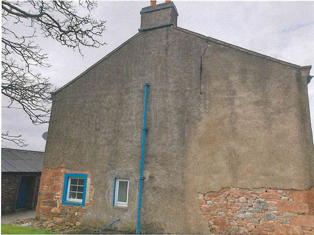
PHOTOGRAPH 03 VIEW ON LEFT HAND GABLE CRACKS
