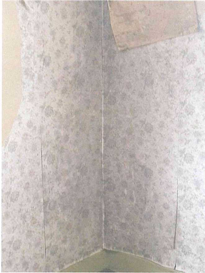
PHOTOGRAPH 05 VIEW ON MILDEW AND DAMP TYPICAL.
