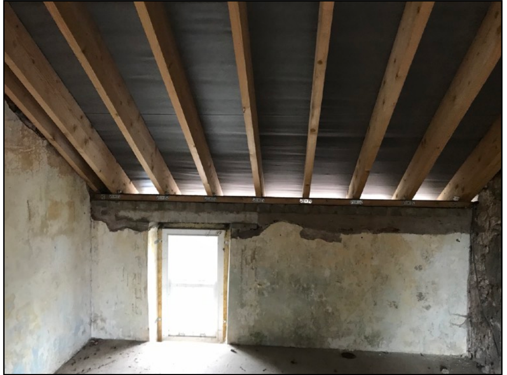
Figure 4: Showing the interior of the farmhouse (First floor) with new roof and unenclosed eaves.
