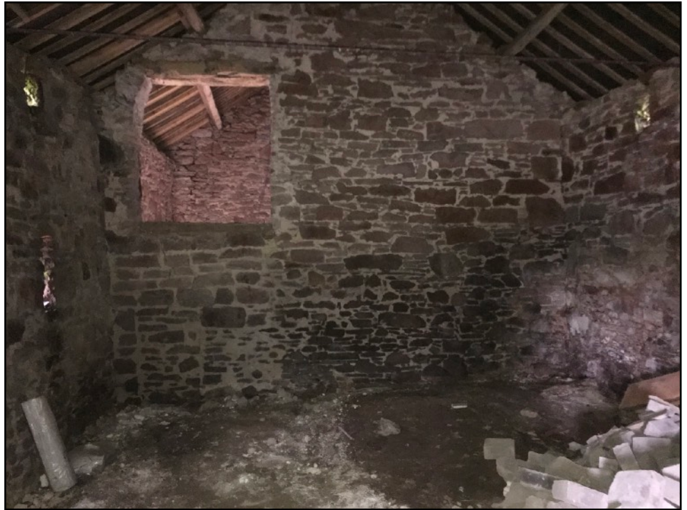
Figure 6: Showing the interior of the barn.
