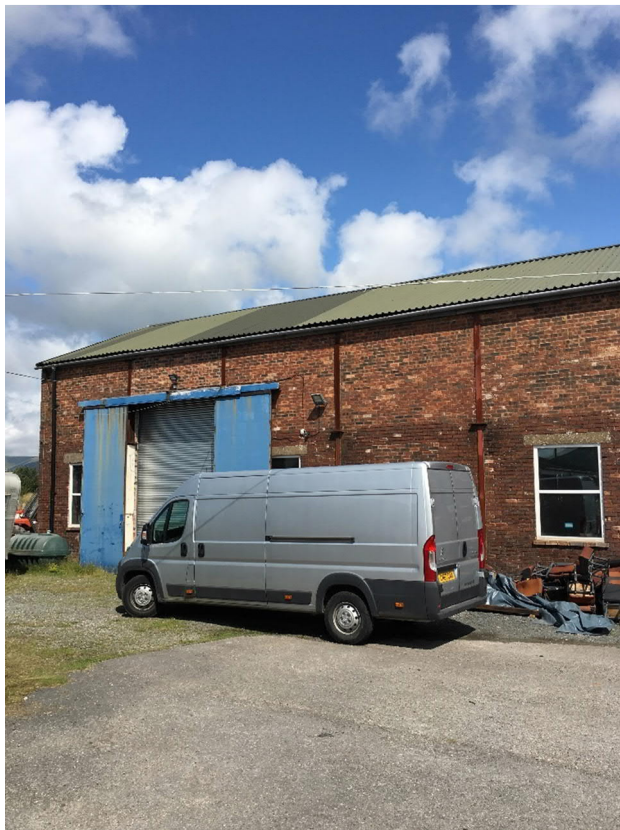
Photograph 6: Warehouse (external – brick built with metal corrugated roof)
