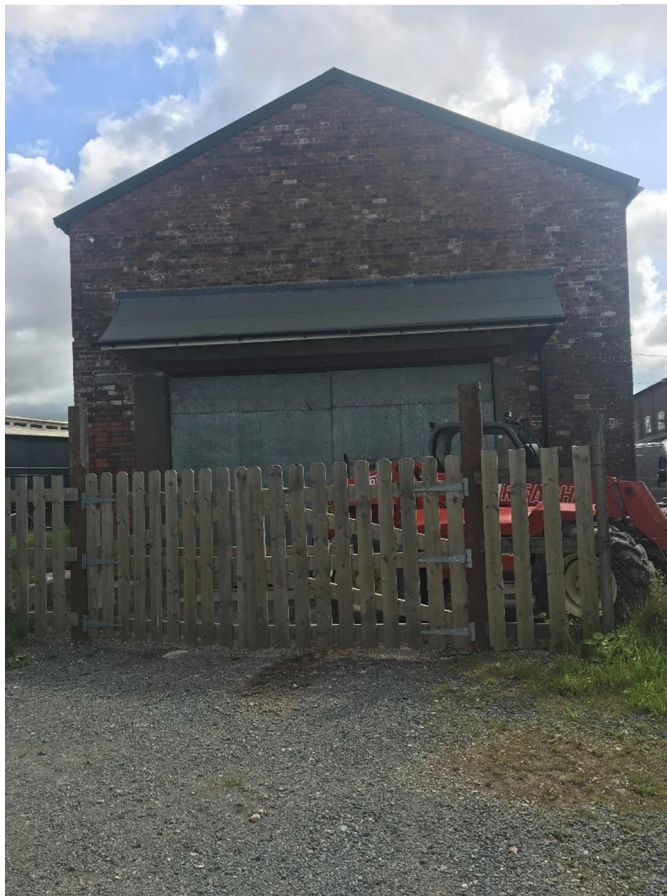
Photograph 18: Gable end of warehouse with plastic enclosed fascia and soffit.
