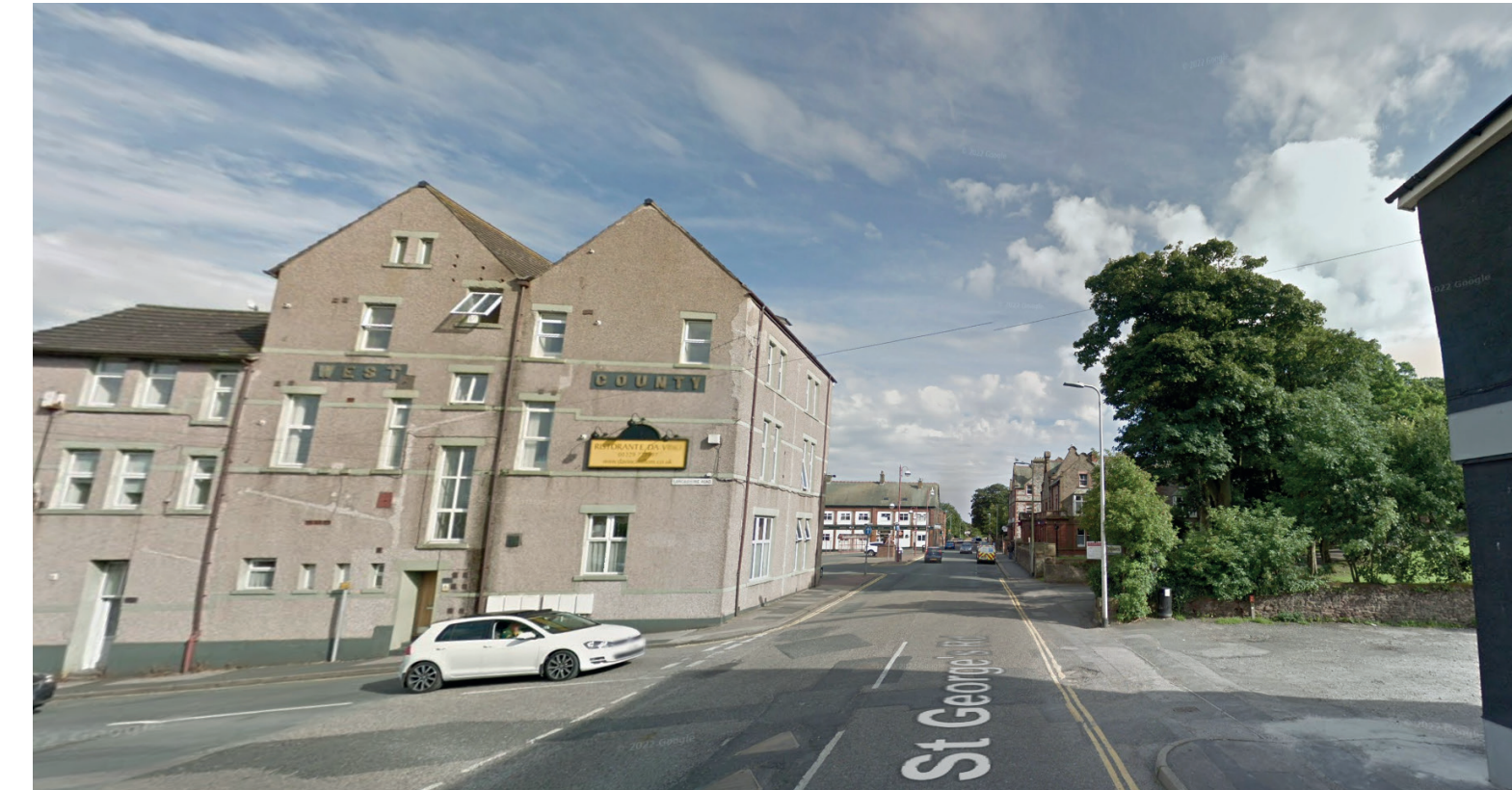
FIG 19 Google Earth - Existing Viewpoint
