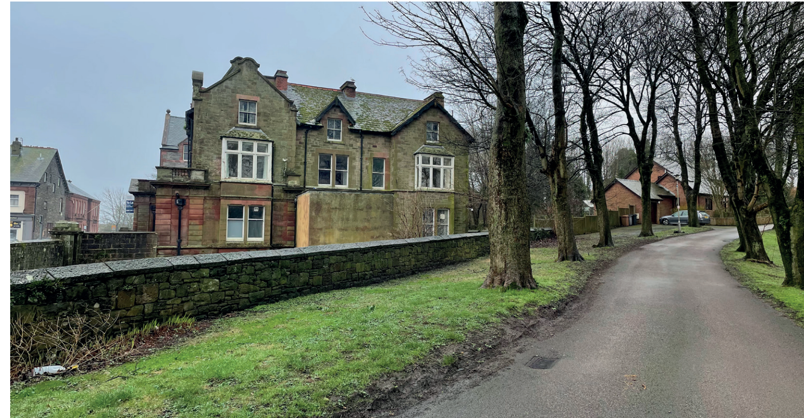
FIG 22 Existing Elevation view from within grounds of Church of St. George.
