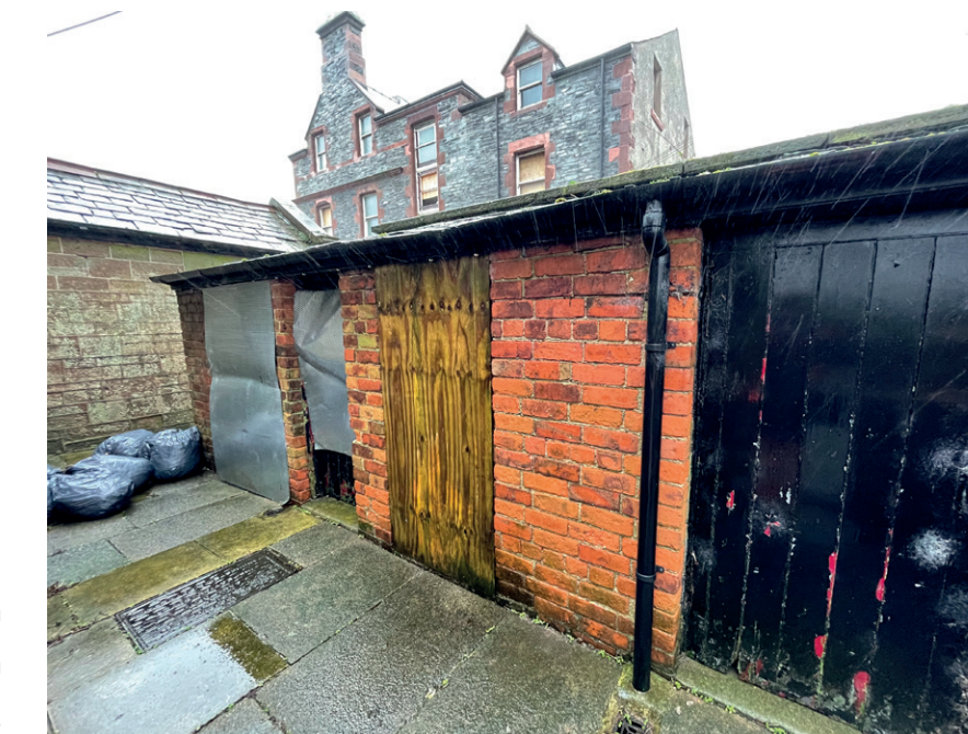
Existing outdoor building retained within garden space to form external work areas for activities such as pottery, and other heavy crafts.
