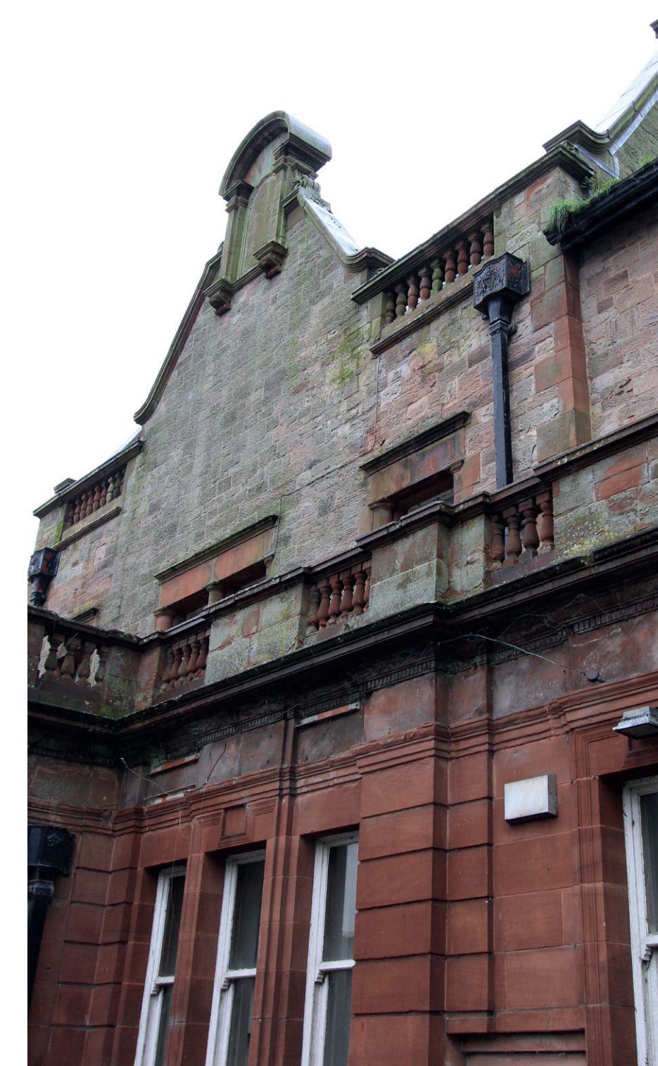
FIG 10 Detail view of Principal Elevation to George St. elevation.
