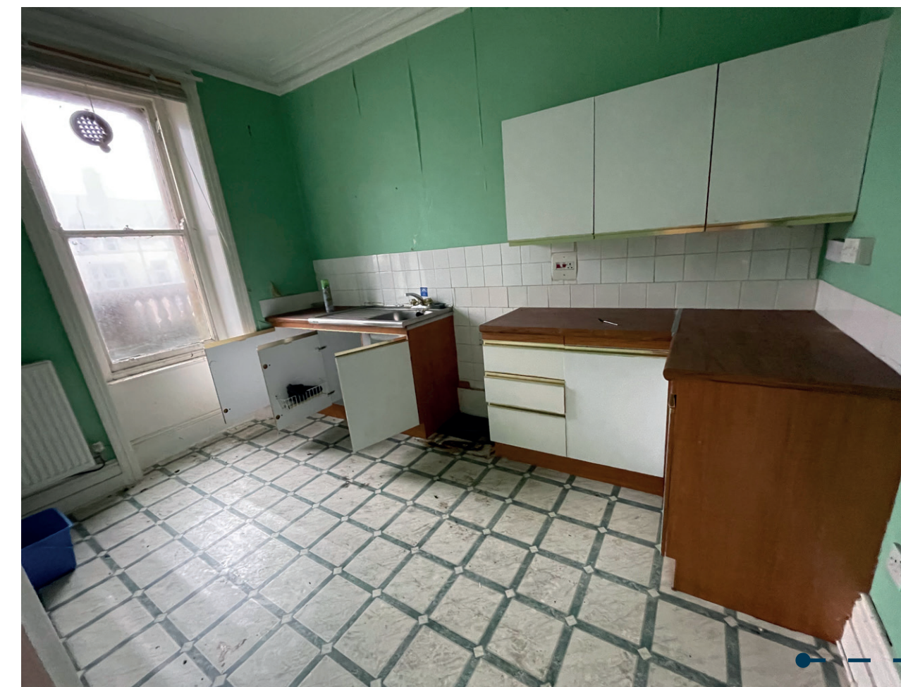
FIG 12 Internal images of former bank building.
