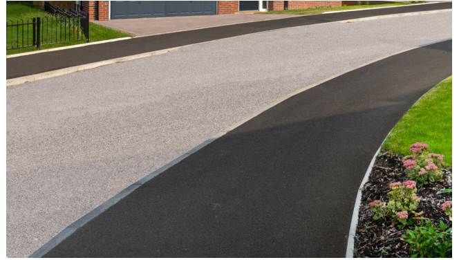
Tarmacadam road & footpath
