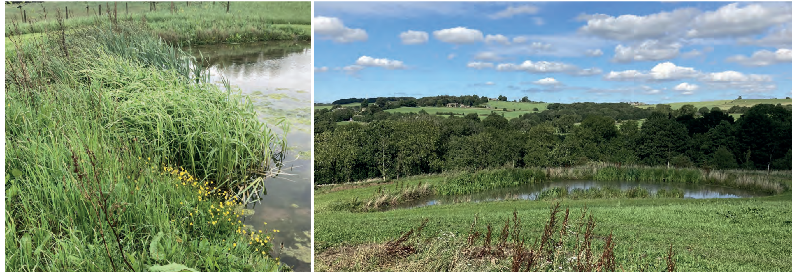
The site has the advantage of space and gradient, two attenuation ponds have been positioned to take surface water and slow the flow into the wider water system. The attenuation ponds would be planted with native, marginal plants and form two rich, wildlife habitats.
