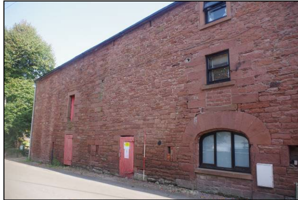
Figure 5. Entrance to a cart shed
