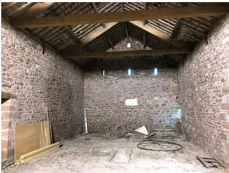
Figure 29. Northern End of Room 4
