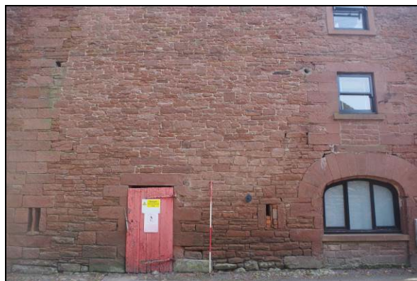
Figure 12. Interface between stone phases
