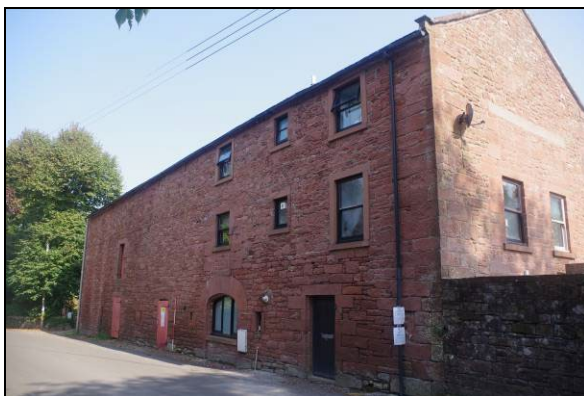
Figure 11. Western elevation with three floors
