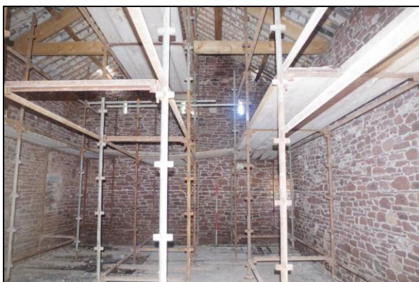
Figure 29. Northern end of Room 4
