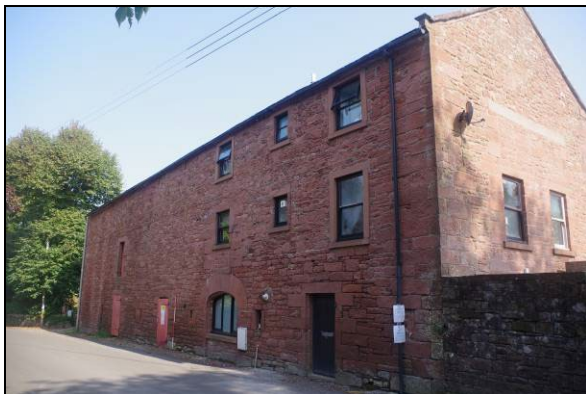
Figure 11. Western elevation with three floors
