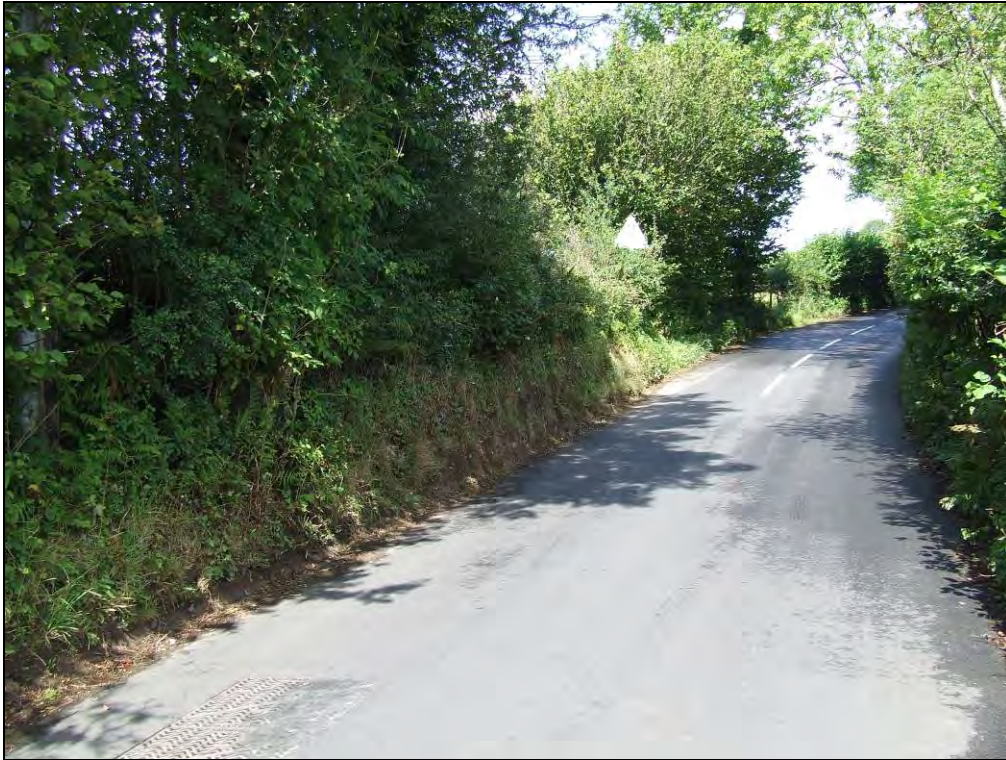
Photo 3: Perimeter – View along the eastern site boundary with Kirkland Road from the south eastern corner of the site, looking north towards the location of the culvert
