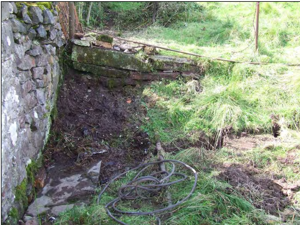
Photo 20: Site Interior – View of small stream channel shown on photo 19, looking west and showing metal pipe crossing path of channel
