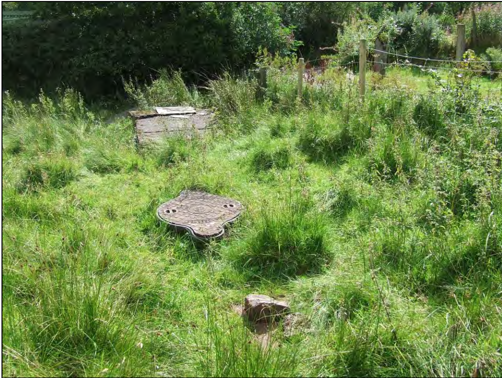
Photo 21: Site Interior – Small private sewage treatment plant located within south western corner of the site with square metal MH cover (foreground), large cast iron MH cover to Klargester (centre) and rectangular brick constructed sump or soakway (top)
