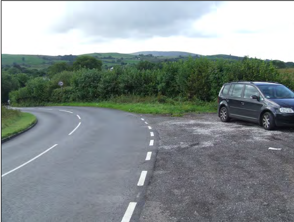
Photo 1: Perimeter – Layby off Kirkland Road adjoining the north eastern corner of the site, looking south west
