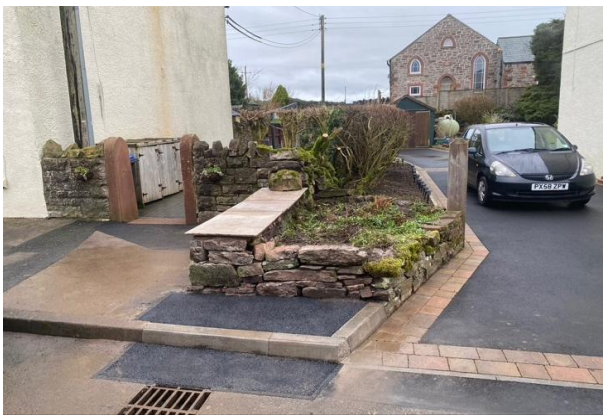
Creation of Vehicular Access & Dropped Kerb (Option 2.0)
