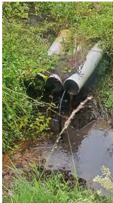
300MM SW OUTFALL INTO BECK
