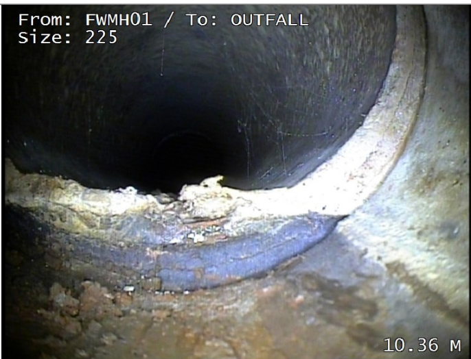
Joint displaced large
