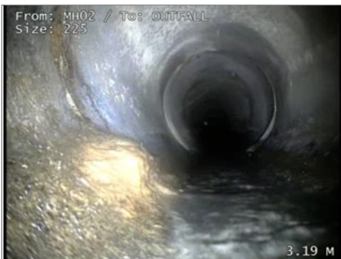
Attached deposits, encrustation at 7 o'clock 5% cross-sectional area loss at joint
