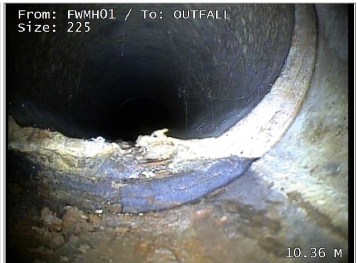
Survey abandoned - Remark: UNABLE TO PASS JOINT
