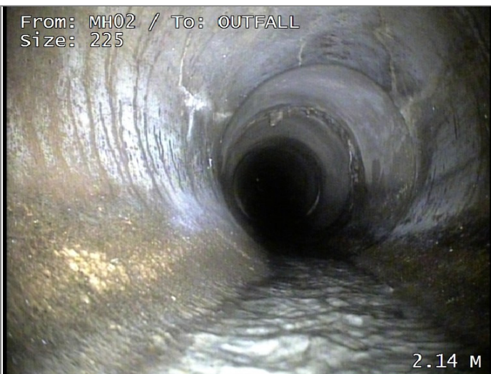
Fracture longitudinal at 10 o'clock
