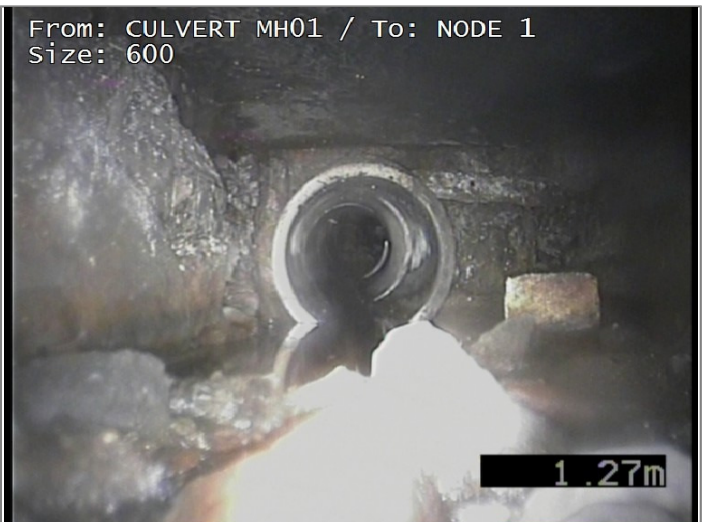
Survey abandoned - Remark: ABANDONED DUE TO DEBRIS
