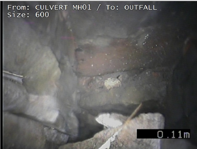
Survey abandoned - Remark: UNABLE TO PASS DEBRIS
