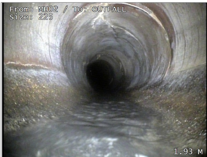
Fracture longitudinal at 12 o'clock, at joint
