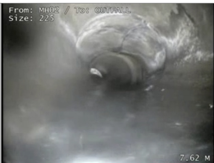
Fracture longitudinal at 12 o'clock
