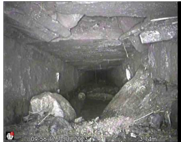
Culvert 1X_18759280-8c50-49a7-812e-a6b0ab322bbd_20230712_15 2834_768.jpg, 00:00:21, 2.36 m Other obstacles, other object in invert from 03 o'clock to 07 o'clock, 30% cross-sectional area loss, displaced stone
