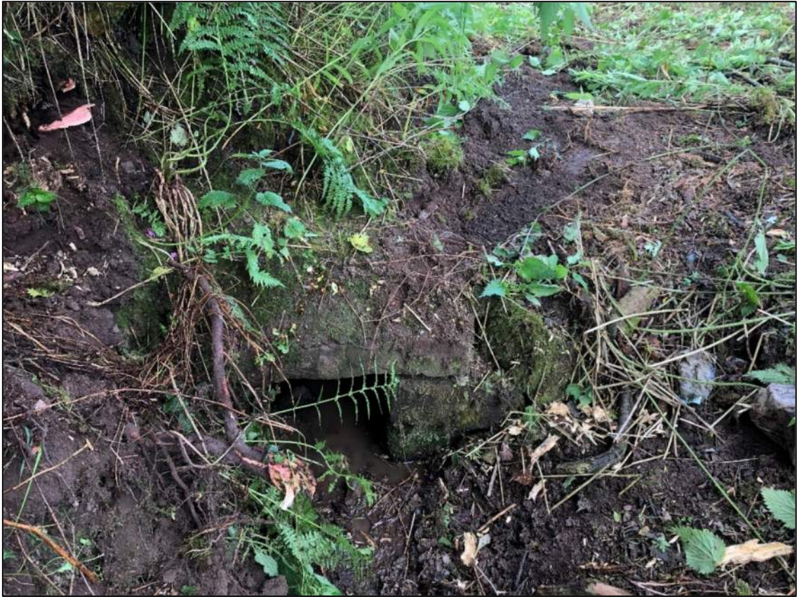
Figure 2.4 Culvert inlet and ditch
