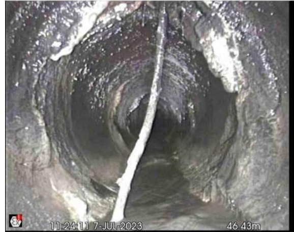
S2X_97c2849a-d9bb-4510-8ab3-7ec4e5bc6d6d_20230712_154840_160.jpg, 00:03:35, 46.43 m Roots, tap
