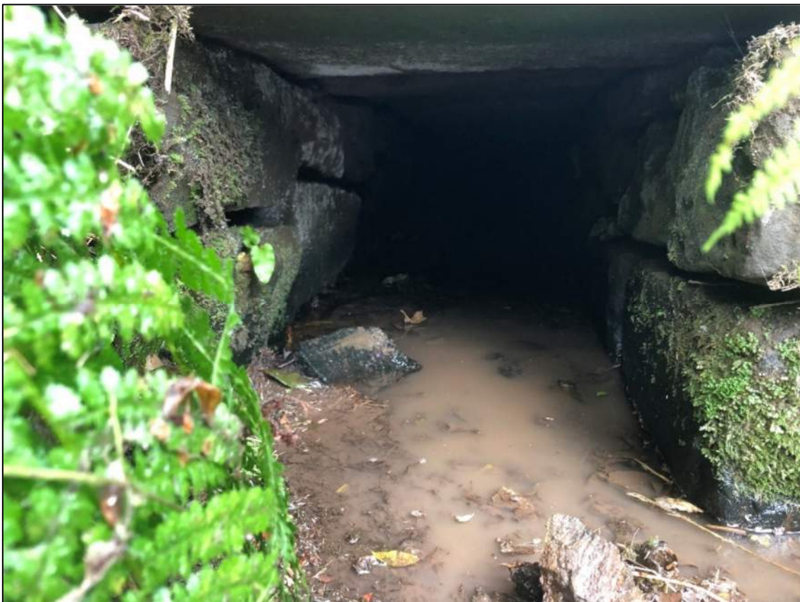
Figure 2.5 View up culvert inlet
