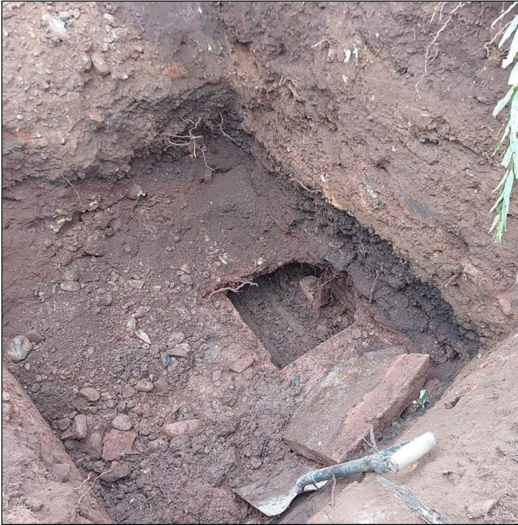
Figure 2.6 Excavation on Culvert at Extent of Camera Survey
