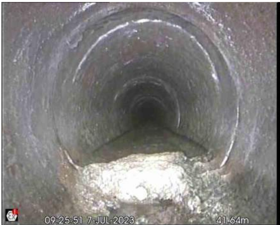
UpstreamX_d0f13ee9-871a-4629-ba44-8d6ef983a3a5_20230712_152448_915.jpg, 00:03:03, 41.64 m Other obstacles, other object in invert from 04 o'clock to 08 o'clock, 25% cross-sectional area loss
