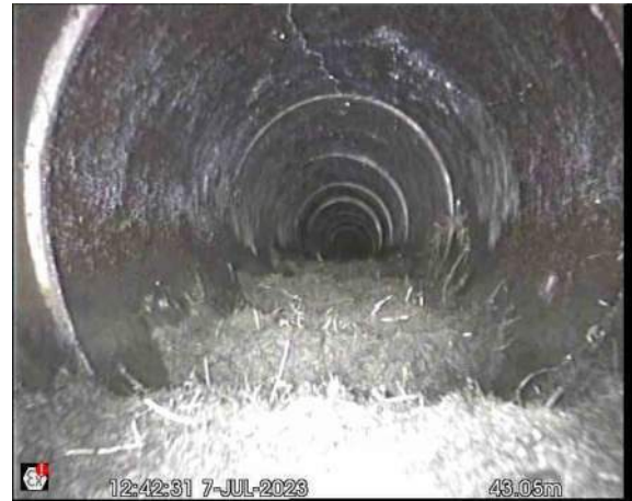
S1X_45acfc27-6d4f-4806-ab6a-398c2d1aa1b4_20230712_153627_751.jpg, 00:02:48, 43.05 m Roots, mass, 20% cross-sectional area loss
