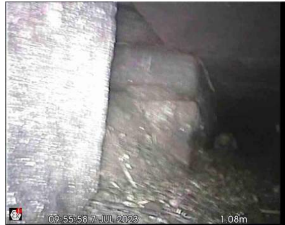
Culvert 1X_1094904e-3591-43dd-b28d-2fe7ede5a29a_20230712_15 3001_075.jpg, 00:00:16, 1.08 m General photograph taken at this point, connecting culvert from the left ???
