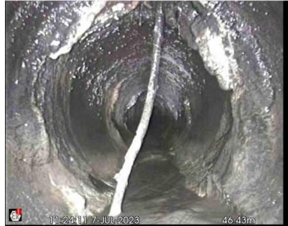
S2X_97c2849a-d9bb-4510-8ab3-7ec4e5bc6d6d_20230712_154840_160.jpg, 00:03:35, 46.43 m Roots, tap
