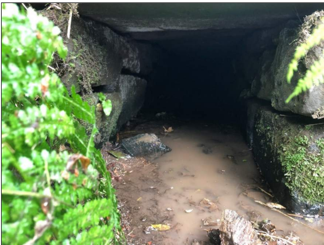
Figure 2.5 View up culvert inlet
