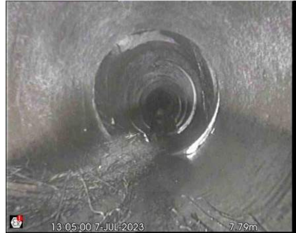
S1aX_83cce470-f0bc-443b-b859-a585f6d0a394_20230712_154244_815.jpg, 00:00:35, 7.80 m Roots, fine
