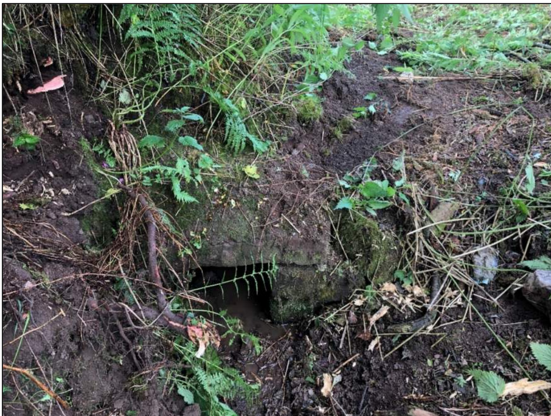
Figure 2.4 Culvert inlet and ditch
