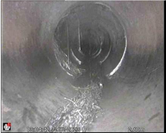
S1aX_9d48a358-d887-4d64-8c53-e56040260046_20230712_154232_072.jpg, 00:00:16, 2.60 m Roots, fine
