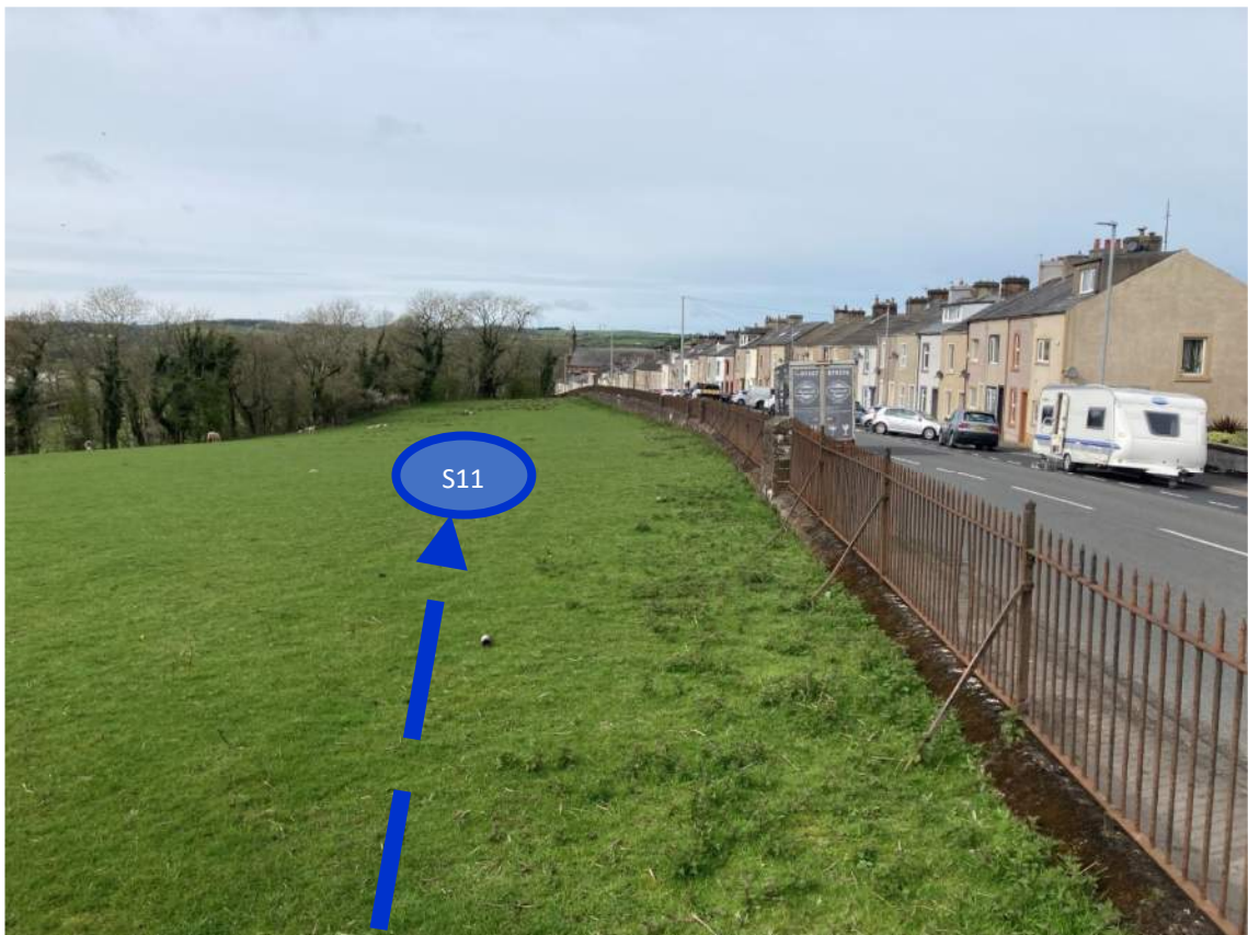
Photo 4 – off-site SW route proceeds south-west, boundary retaining wall tapers down
