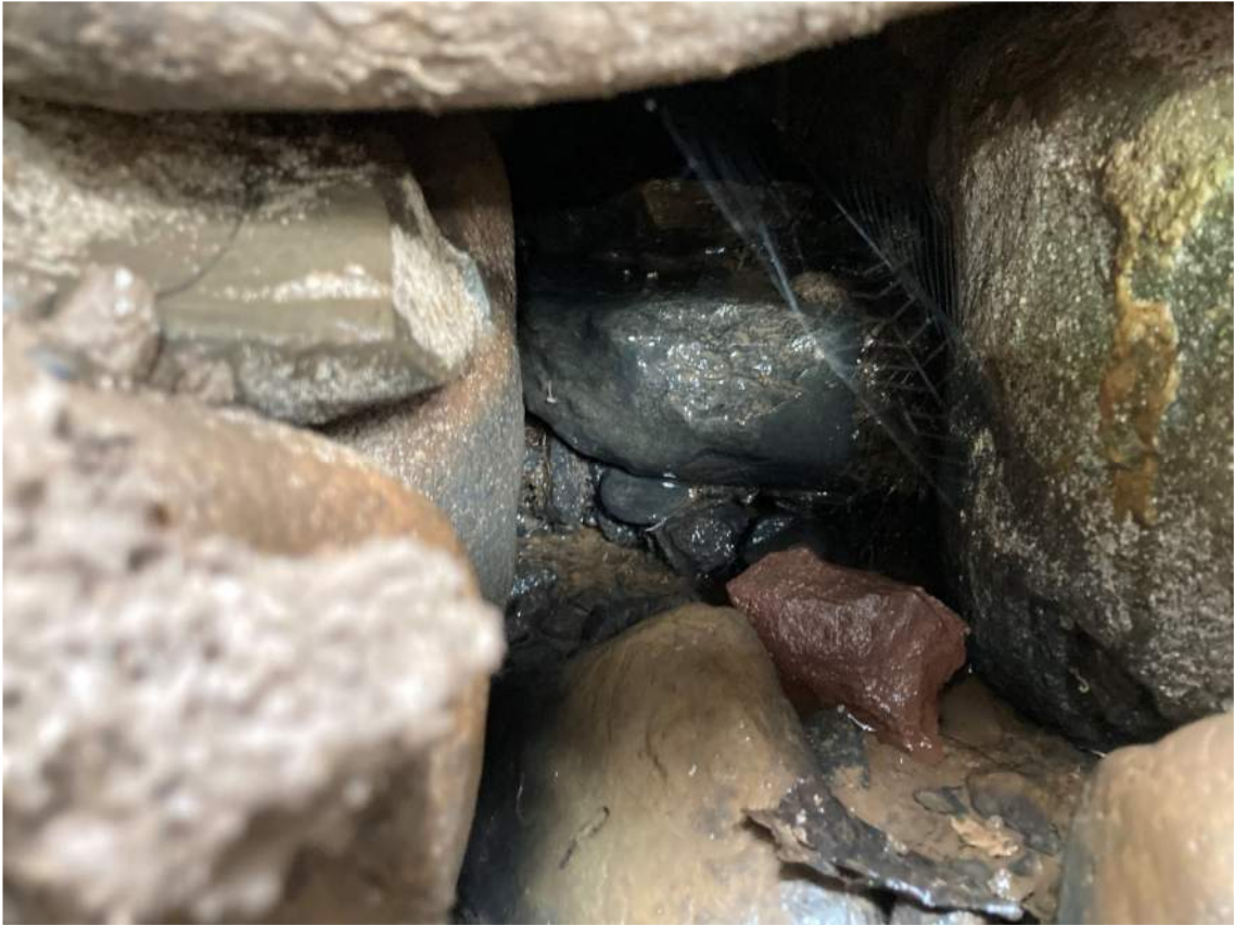
Photo 7 – existing stone culvert land drainage outfall
