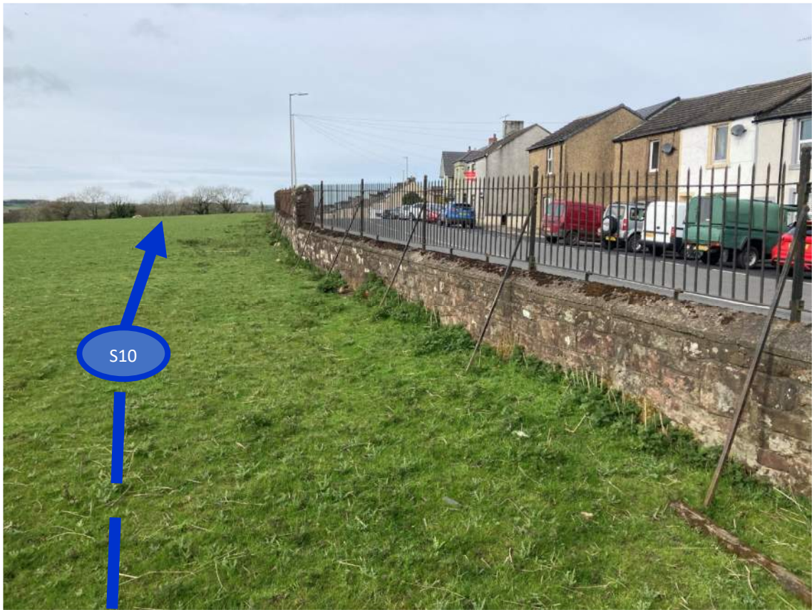
Photo 3 – off-site SW route running south-west parallel to boundary retaining wall (6 – 8m from wall)
