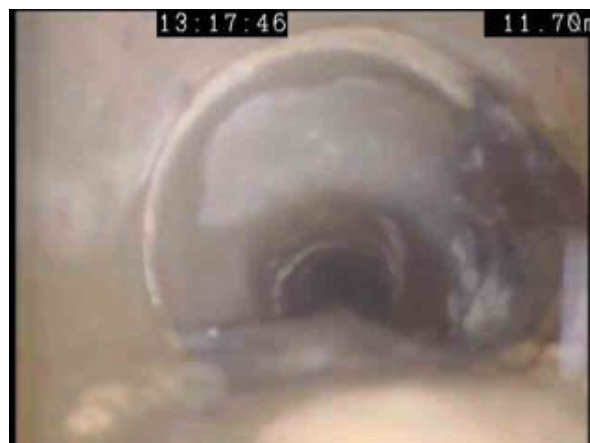
MH1X_30e8334b-3829-497f-ab2e-a0ecc3aaf3e5_20200225_152335_298.jpg, 00:01:25, 11.70 m Attached deposits, encrustation at joint from 02 o'clock to 06 o'clock, 10% cross-sectional area loss
