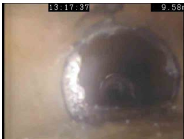
MH1X_10743e70-1bdd-4d25-af42-1f804335d3ec_20200225_152256_324.jpg, 00:01:16, 9.58 m Attached deposits, encrustation at joint from 12 o'clock to 12 o'clock, 10% cross-sectional area loss
