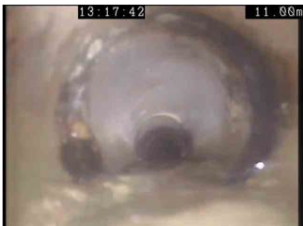
MH1X_d09dd2a7-3195-485d-a33c-282457107e09_20200225_152318_902.jpg, 00:01:22, 11.00 m Attached deposits, encrustation at joint from 12 o'clock to 12 o'clock, 5% cross-sectional area loss
