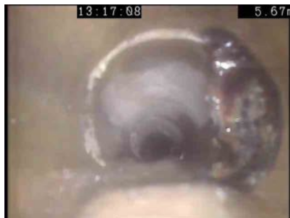
MH1X_53f2d50c-f3e5-431f-b108-4a90485e6efe_20200225_152004_133.jpg, 00:00:47, 5.67 m Attached deposits, encrustation at joint from 01 o'clock to 06 o'clock, 20% cross-sectional area loss
