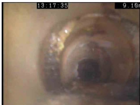
MH1X_f37de10b-7df3-403f-99df-838bb01db9db_20200225_152216_384.jpg, 00:01:14, 9.10 m Attached deposits, encrustation at joint from 12 o'clock to 12 o'clock, 10% cross-sectional area loss
