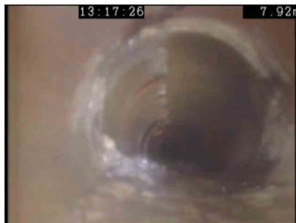
MH1X_48eec4de-904f-4be5-ba33-f21f81524477_20200225_152140_366.jpg, 00:01:05, 7.92 m Attached deposits, encrustation at joint from 02 o'clock to 09 o'clock, 15% cross-sectional area loss
