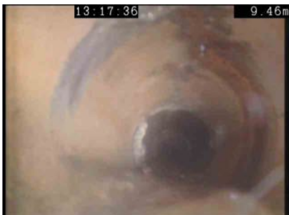
MH1X_7ed44ac0-38be-47e1-a4fb-6f627d3fb9fa_20200225_152240_818.jpg, 00:01:15, 9.46 m Crack, longitudinal at 12 o'clock
