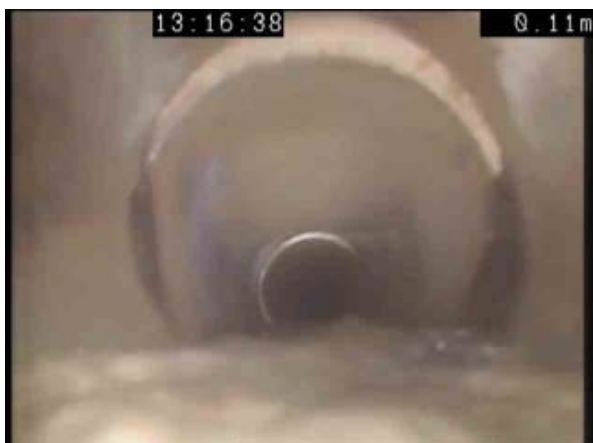
MH1X_e82f07f4-4278-4096-a40b-4d0c8a52a017_20200225_151916_131.jpg, 00:00:18, 0.12 m Joint displaced, medium
