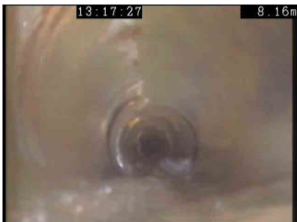
MH1X_60aa83a6-cc65-408f-b89e-f3a013ebb865_20200225_152153_002.jpg, 00:01:06, 8.16 m Crack, longitudinal at 11 o'clock
