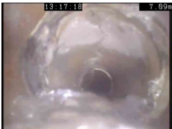
MH1X_6d548981-5f12-419a-b0c6-33c25c06ac12_20200225_152045_590.jpg, 00:00:57, 6.97 m Attached deposits, encrustation at joint from 12 o'clock to 12 o'clock, 5% cross-sectional area loss
