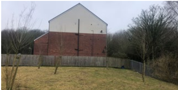
2. View west showing blank gable from existing flats.
