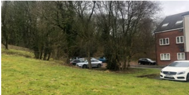
7. View north west showing existing parking court and trees.
