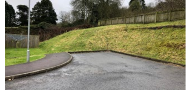
9. View of south west corner, level change and turning head.
