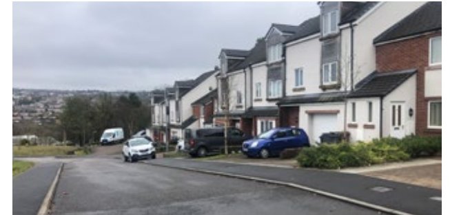
12. View east showing existing private road and houses.
