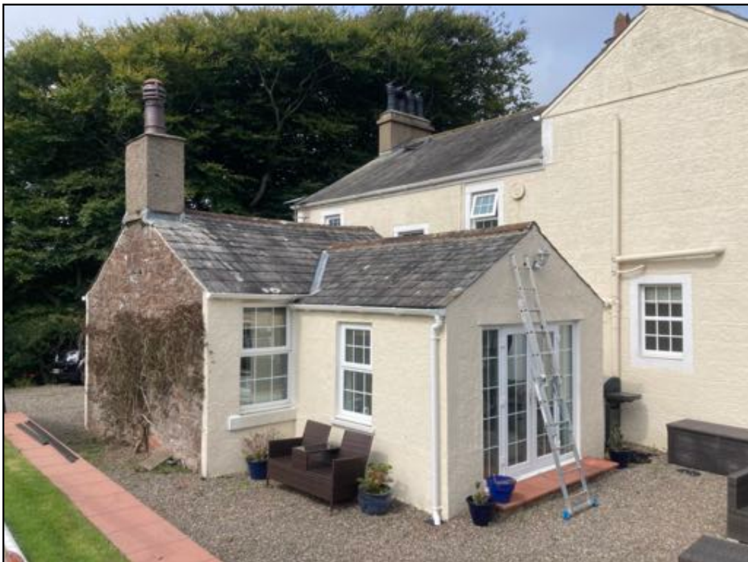
Figure 5: Showing the kitchen sections from the southwest - slate clad roof and ridges - very tightly set, despite a through search from ladder height, there was no typically suitable access for bats present.
