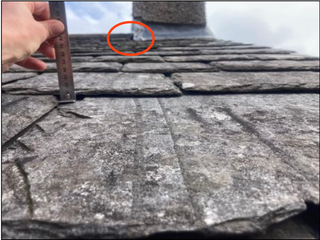
Figure 4: Showing minimal / unlikely gaps for bats throughout the kitchen roof - there was a single gap in the flashing at the western pitch - as shown above - that could possibly provide a sub-optimal spaces for a single pipistrelle bat.
