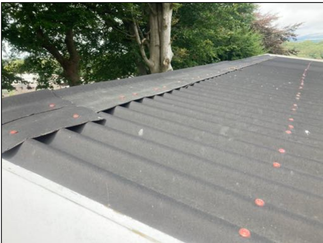
Figure 7: Garage roof - the building is purpose built and the roof has no suitable access for bats and wall tops also do not present gaps or access to suitable voids / crevices. Once the garage here is removed then the trees shown here at the west of the house would be an ideal location to erect bats boxes / bird boxes and enhance the site for bats / birds - if desired.
