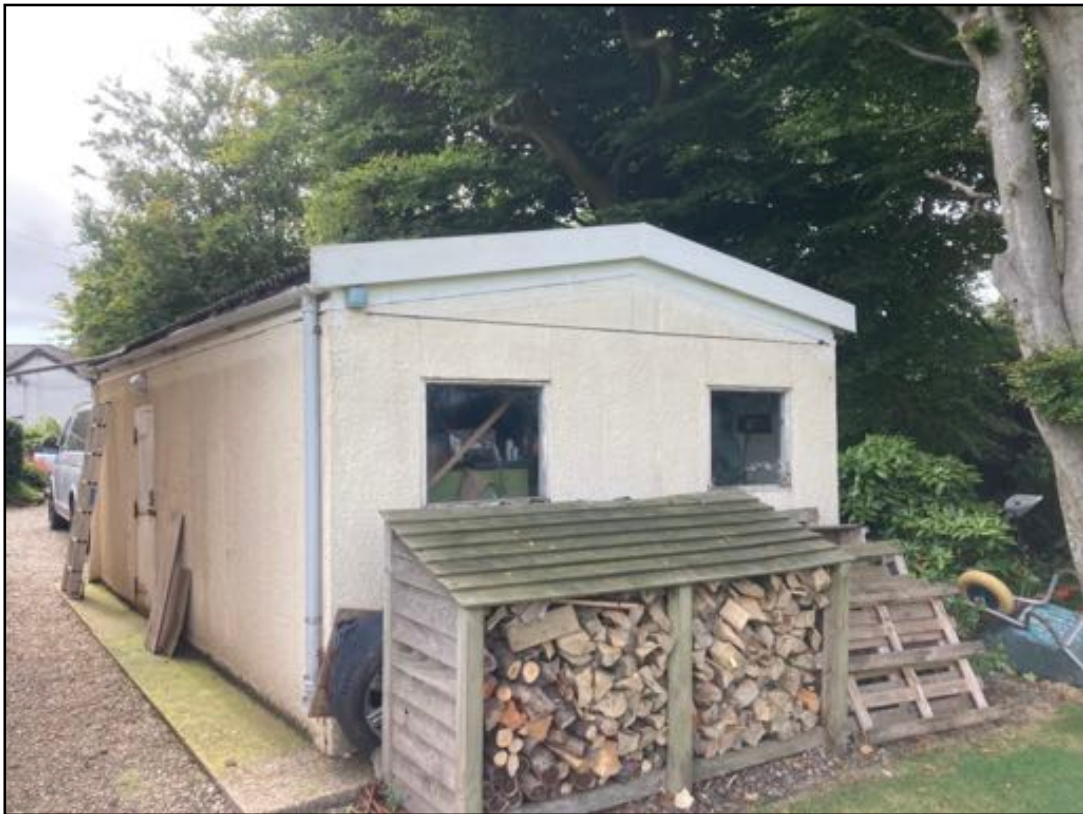
Figure 6: Garage from the north - there were no gaps in the walls and no bat roost potential. The building was generally inaccessible to birds also - there may be some potential for access in gaps above the doors / at the sides at the southern end.
