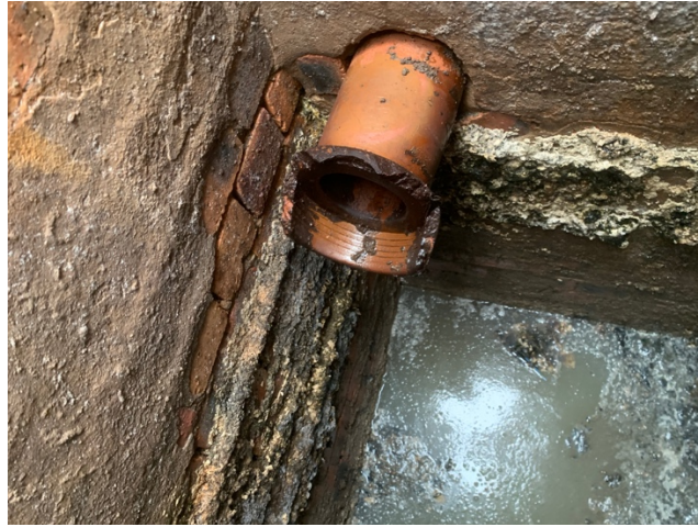
Fig 6. Leak from the outer wall.
