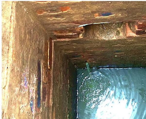
Fig 6. Leak from the outer wall.
