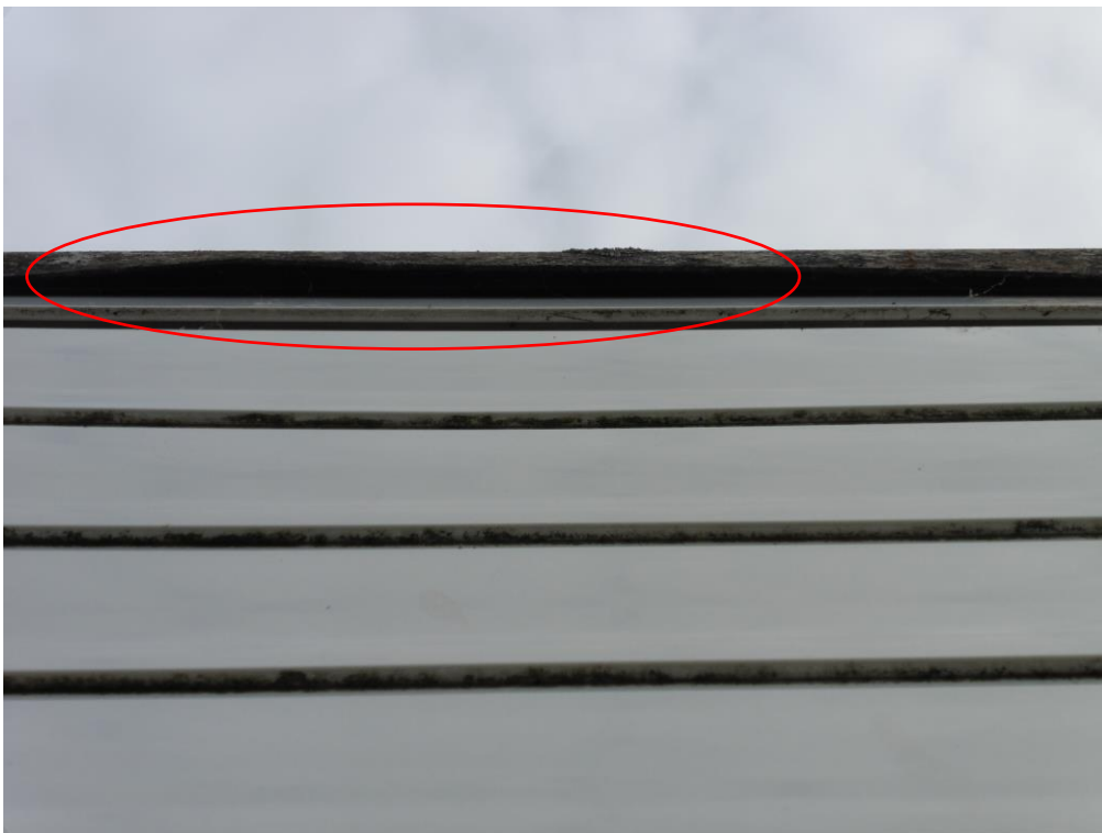
Image 10. Lifted overhanging felt on the southern aspect of F5/F6.
