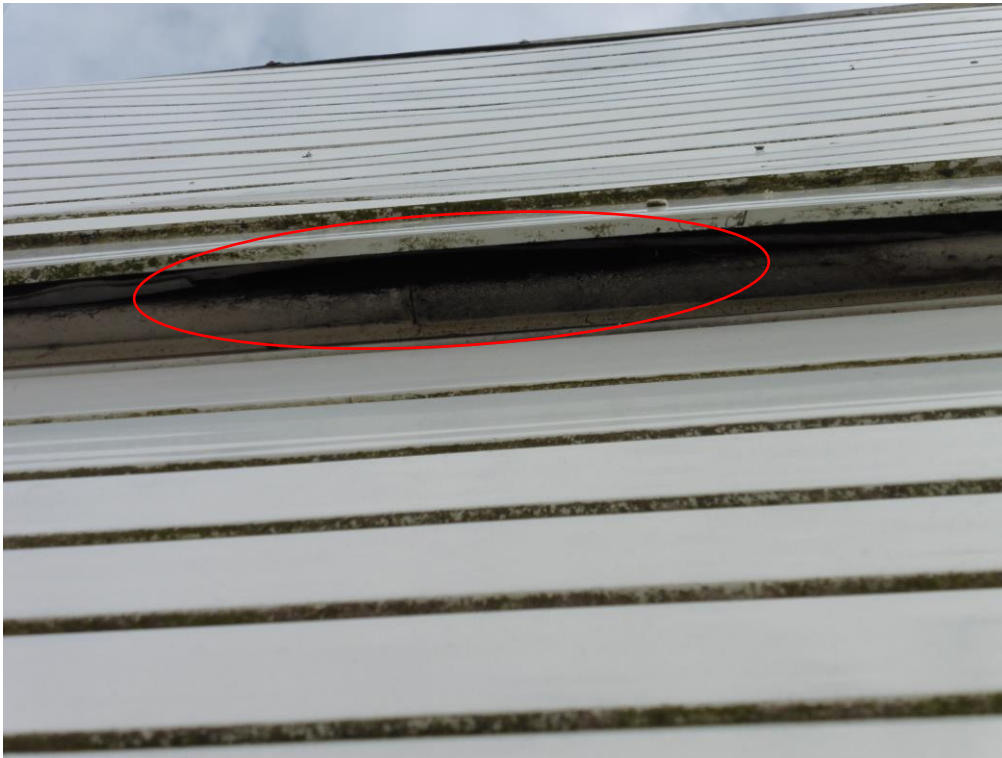
Image 11. Lifted cladding between the two storeys of F5/F6.
