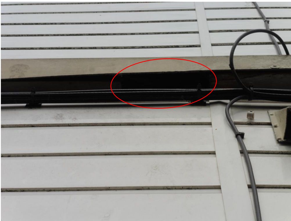
Image 12. Gap within boarding on the eastern aspect of F5/F6.
