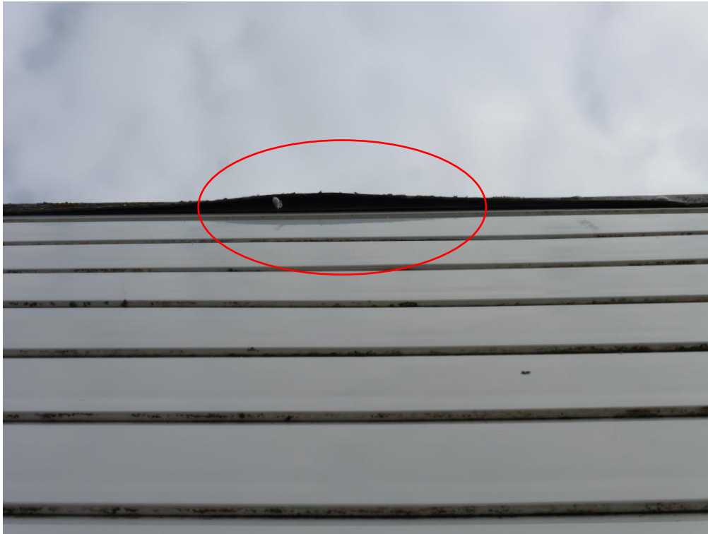
Image 5. Lifted overhanging felt on the southern aspect of F3/F4.
