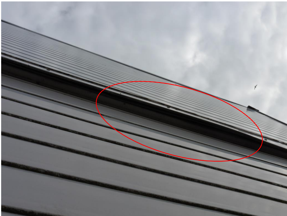
Image 6. Lifted cladding between the two storeys of F3/F4.
