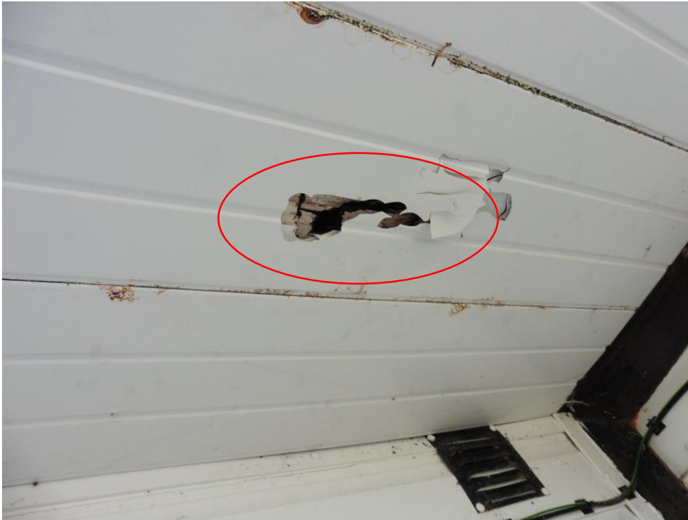
Image 7. Hole above the porch area of F3/F4.
