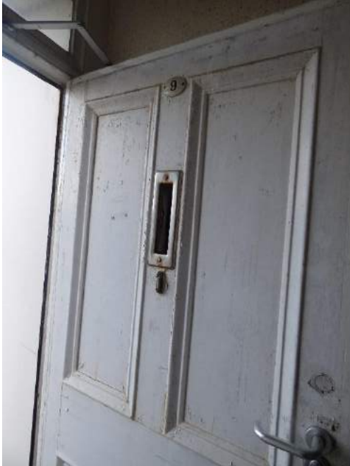
Left and below: Existing door and fanlight to be carefully restored and redecorated.
