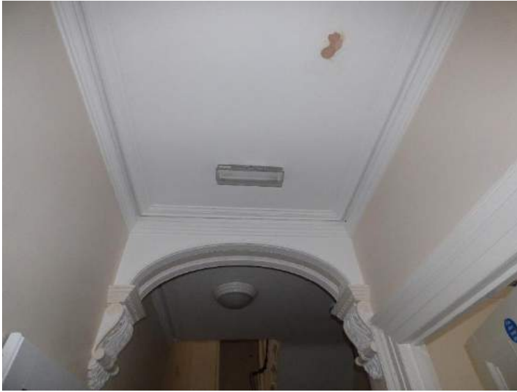
Left: Cornices, architraves and skirtings all in good condition and to be retained.
