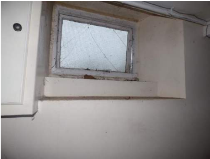
Left: Existing window to be replaced with new slimline double glazed heritage style window with top hinged casement as existing style.
