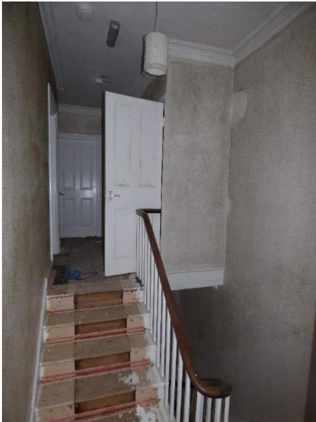
Left: Handrail, balusters and rails are original and are to be retained.
