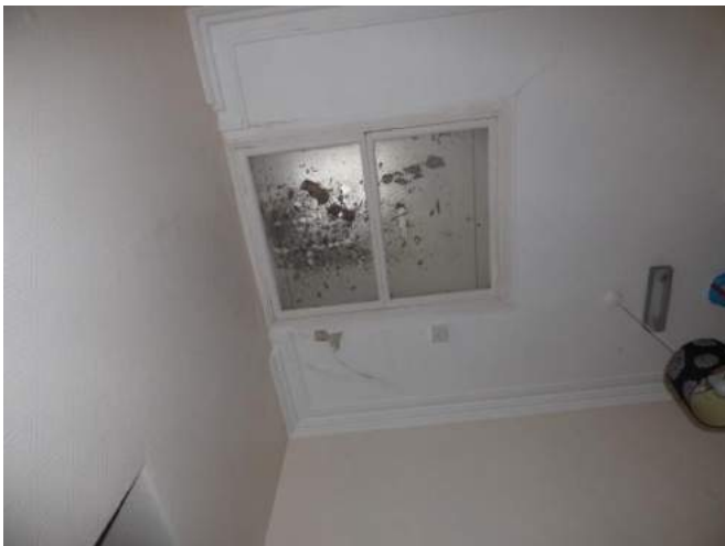
Left: Ceiling glass to be removed and ceiling to be boarded up and cornice to be reinstated where it has been cut out to form glazed aperture.
