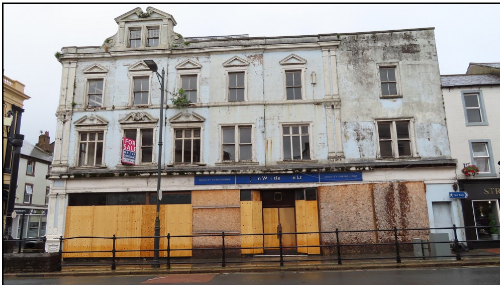
6. The elevation onto Duke Street showing the three phases of development from 1889 to mid 1960's
