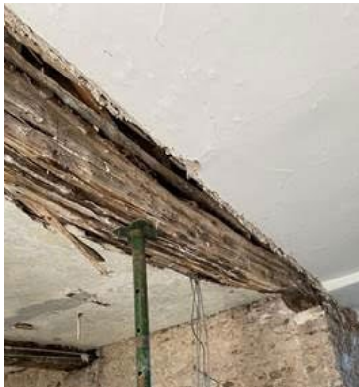
Plates 5 and 6. Details of the original wall beam between kitchen & the entrance hall after removal
