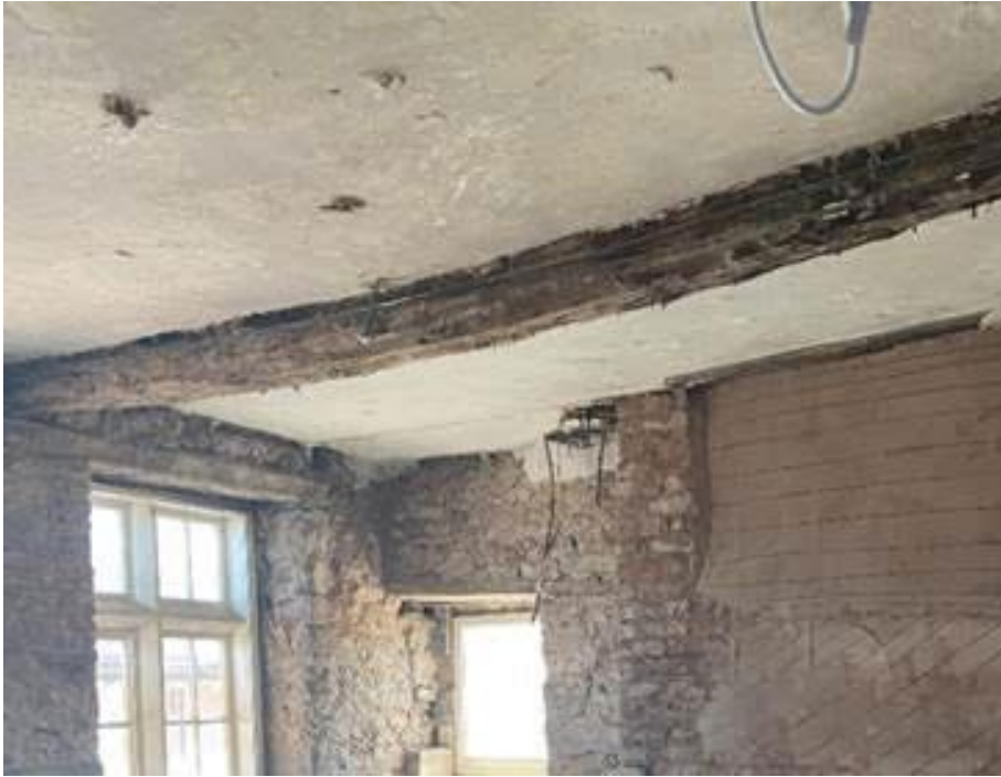
Plate 7. General view of the original wall beam between kitchen & the entrance hall after removal
