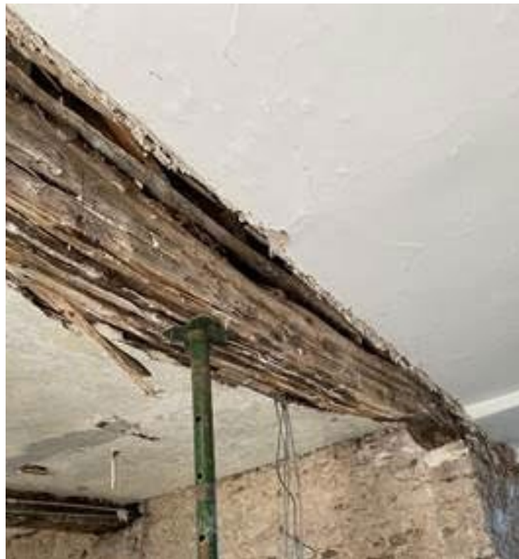
Plates 5 and 6. Details of the original wall beam between kitchen & the entrance hall after removal
