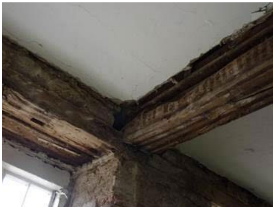
Plates 3 and 4. Details of the original wall beam between kitchen and the entrance hall after removal
