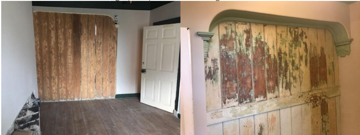
Plates 8-9: Photographs of the front and rear room, ground floor
