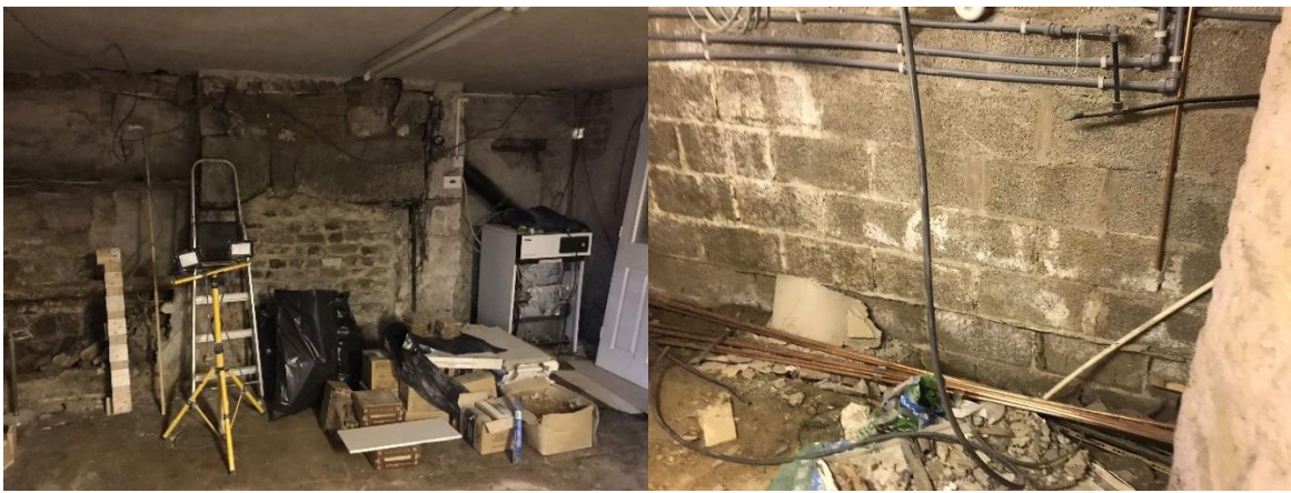
Plates 2-3: Photographs of the basement with flagstone floor and areas of breezeblock wall
