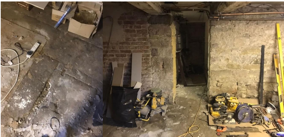
Plates 4-5: Photographs of the basement with historic flagstone floor and areas of historic stone/ brick walling. Note: the timbers overhead have chamfered beams with ogee stops.
