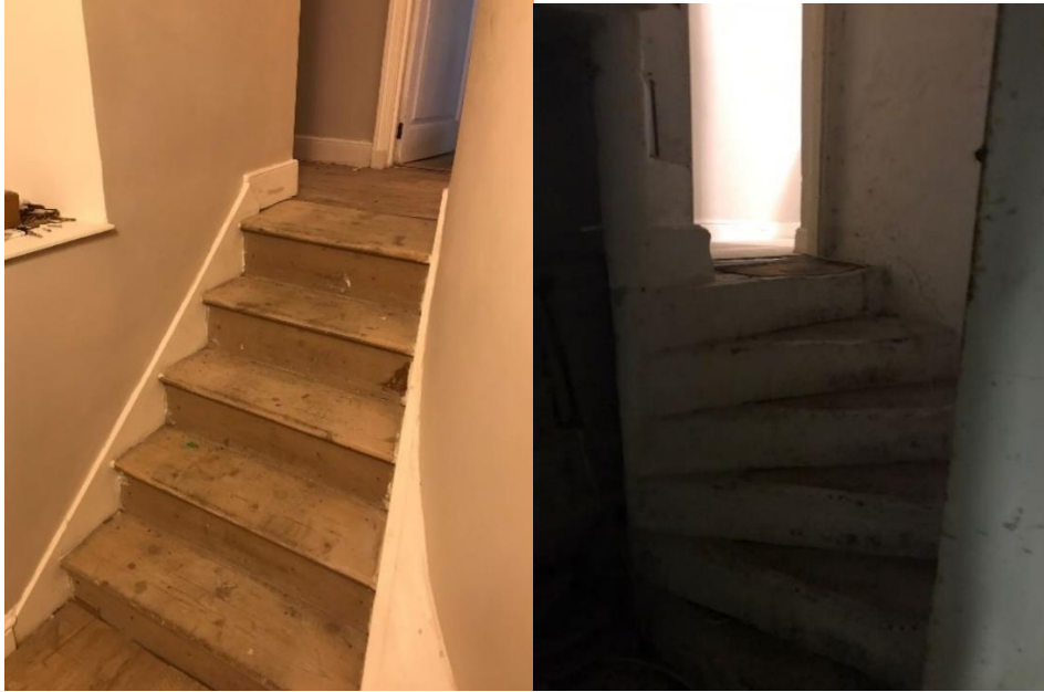
Plates 6-7: Photographs of the staircase at ground/ basement levels
