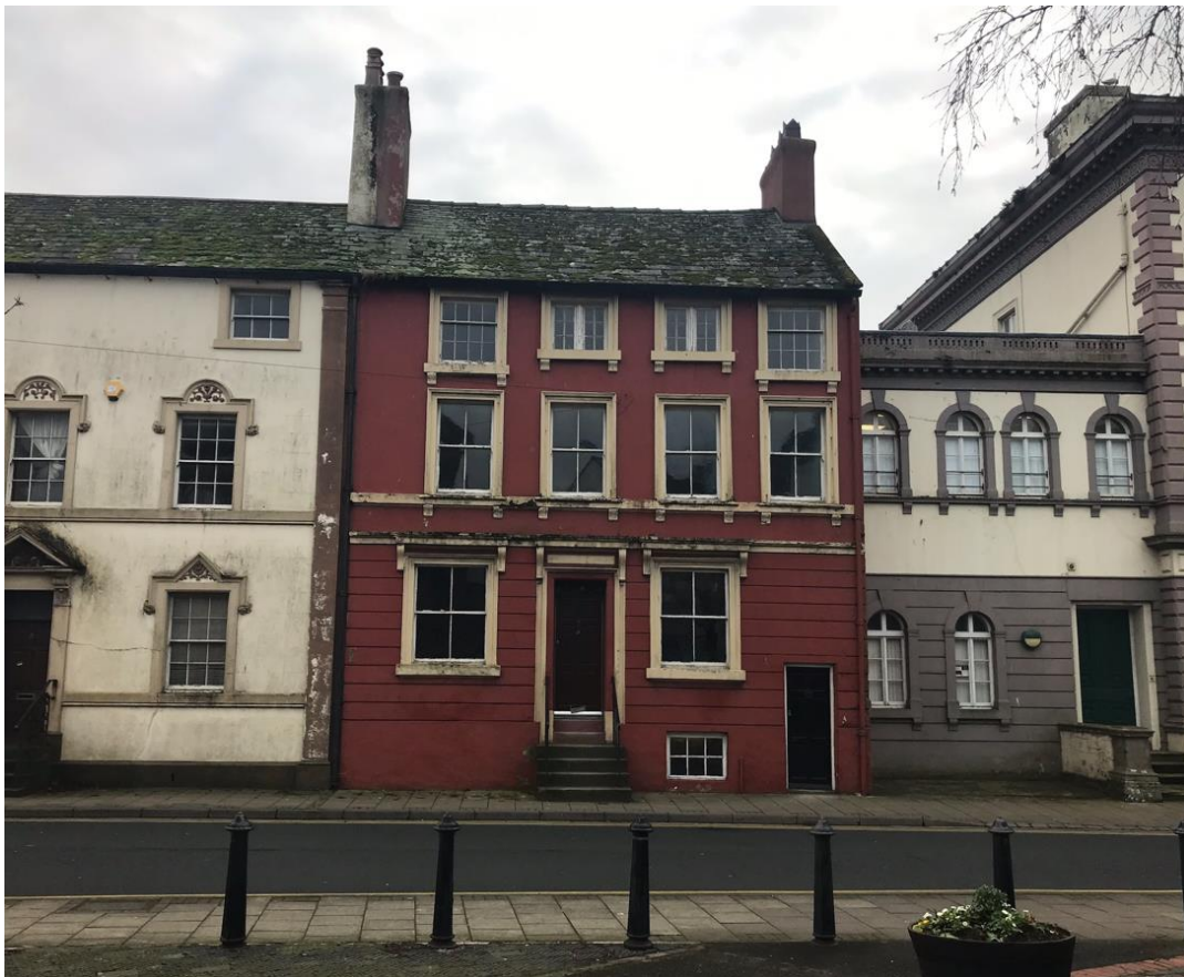
Plate 1: Photograph of the front elevation of 18 Irish Street, Whitehaven January 2023
