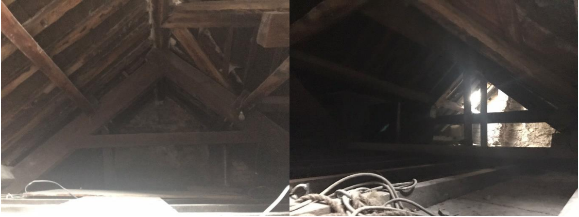
Plates 23-24: Photographs of the roof structure, attic level
