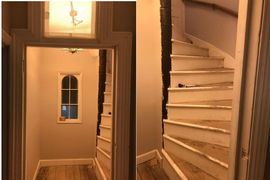
Plates 12-13: Photographs of the staircase at ground/first floor
