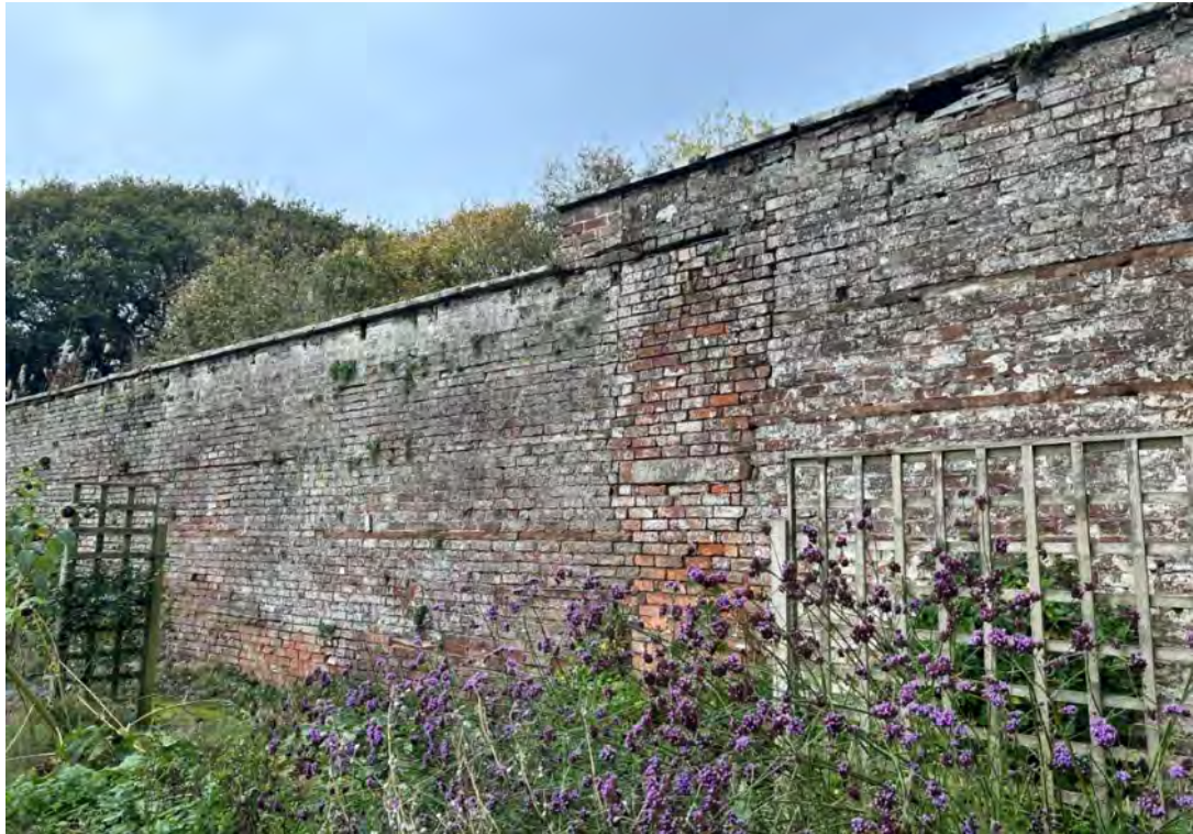
Plate 9, View north towards the northern wall of the garden, the rows of bricks which make up the heating system can be seen within the brickwork,
