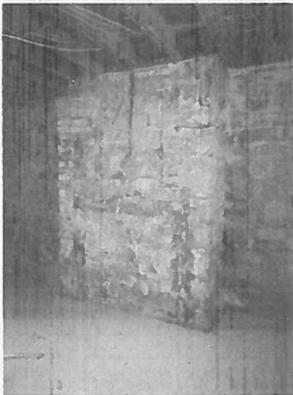
d. Chimney breast to be removed and replaced by B4 in engineers specification
