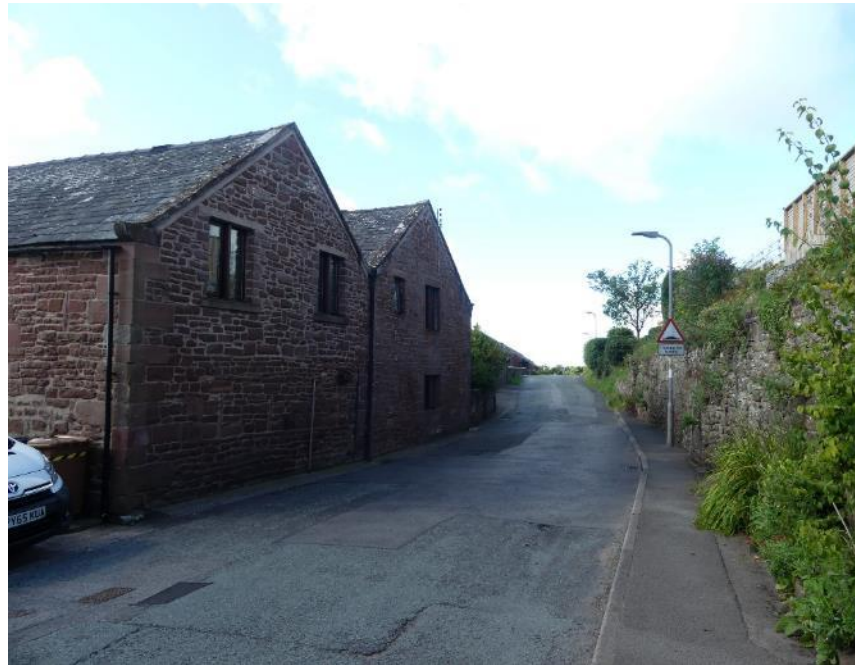
Figure 4.21: The application site is obscured by the landform and alignment of Abbey Road to the west of the Abbey Farm group
