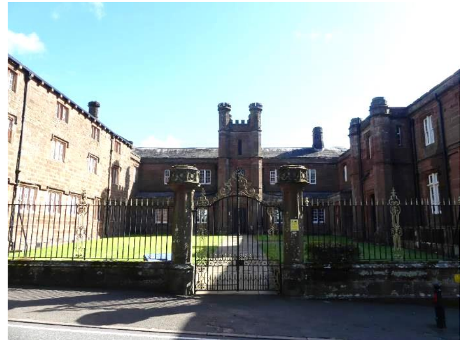
Figure 4.17: The Quadrangle of St. Bees School, with the clock tower aligned with the octagonal gate piers and the north range, considered to be the earliest part of the school, to the left
