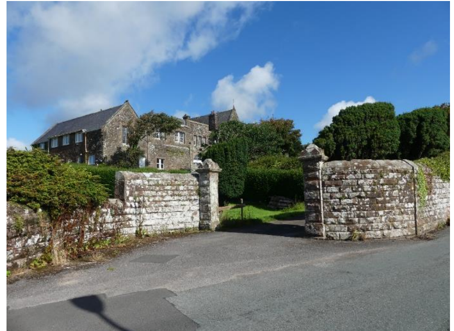
Figure 4.33: The gateway and boundary wall to Abbots Court with the 1930s infill between the two gables
