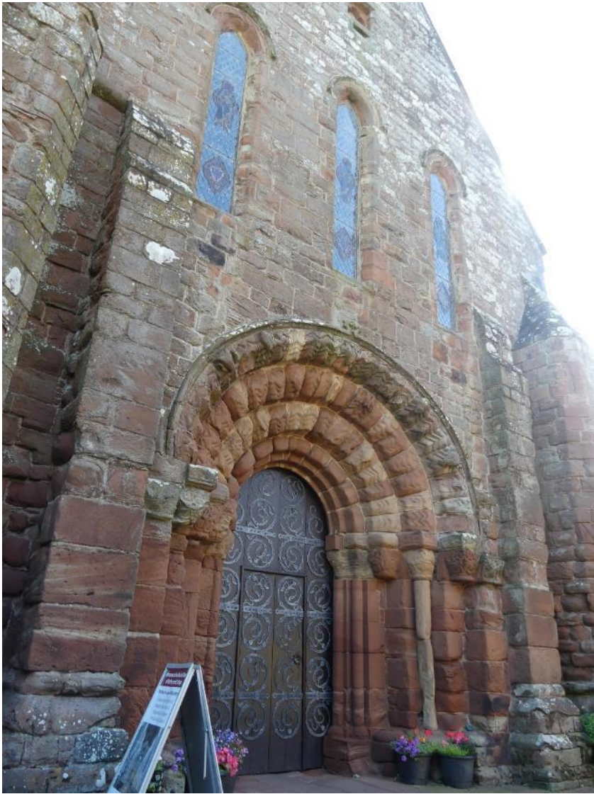
Figure 4.1: The west door with lancets above
