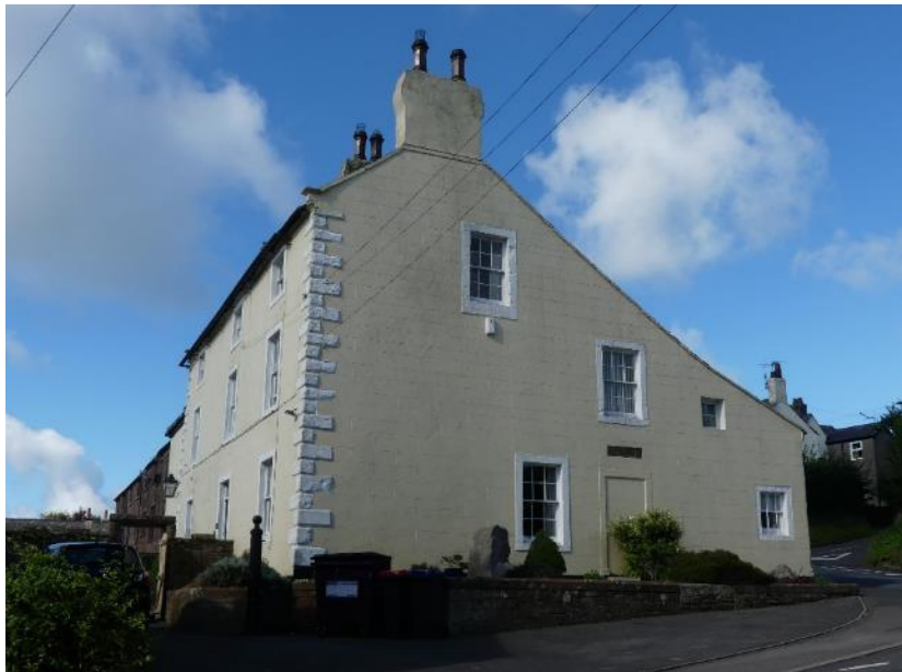
Figure 4.19: The eastern gable and south front of Abbey Farmhouse
