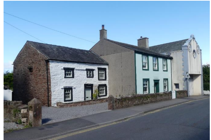
Figure 4.25: The C17th Cottage in the northern part of Main Street
