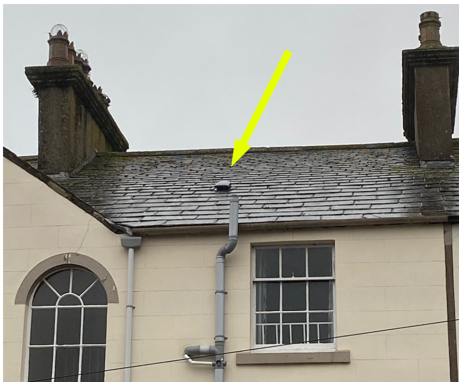
An identical type of slate vent already in place on the main roof of the property.
