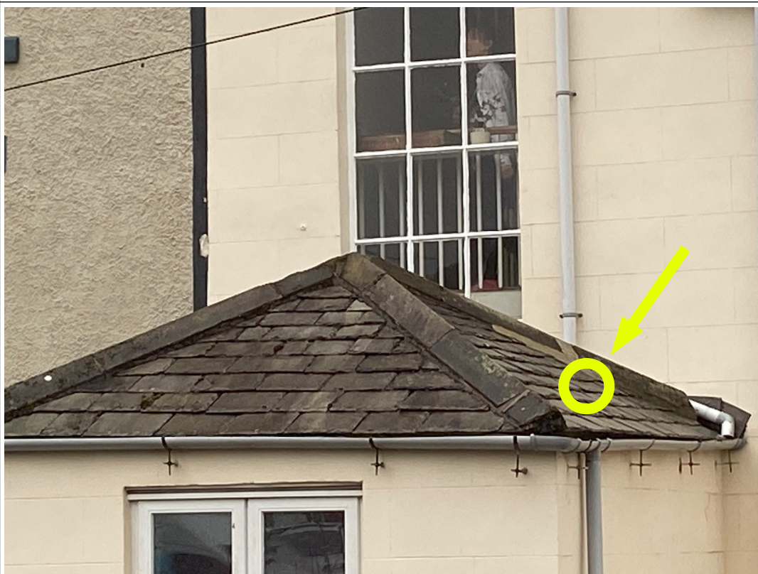
View of the rear offshoot. The approximate location of the new slate vent is indicated.
