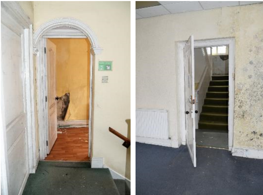
Figure 29 & 30 – internal photograph showing 2no. stairwell doors to be blocked up.
