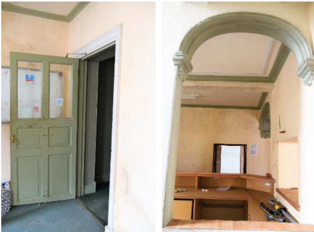
Figure 20 & 21 – internal photograph showing living room door and kitchen hatch to be blocked up.
