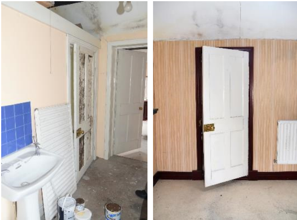
Figure 34 & 35 – images showing 2no. doors to the stairwell to be blocked up.
