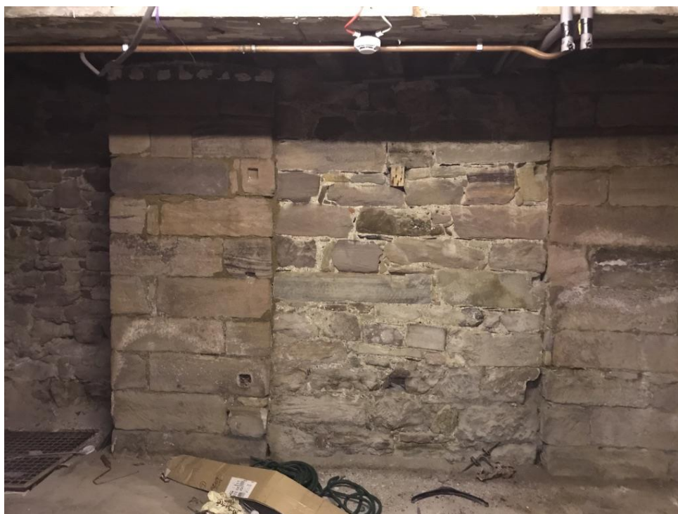
Basement area under the main building
