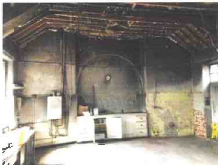
Fig 14 below, main kitchen area which has been destroyed due to a fire
