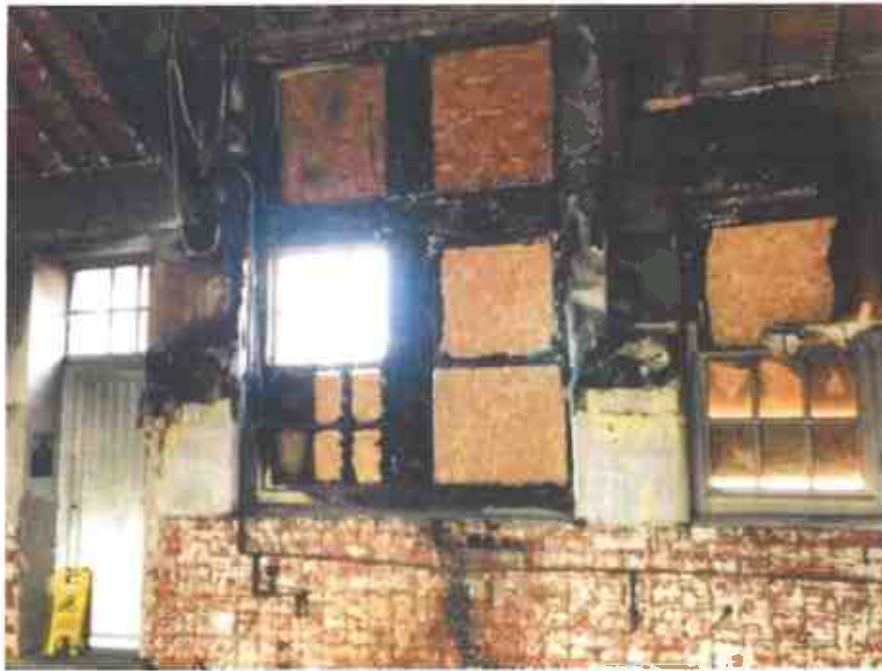
Fig 15 Kitchen area main windows and roof which will need replacement.
