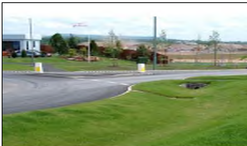
Photo showing edge of carriageway detail
