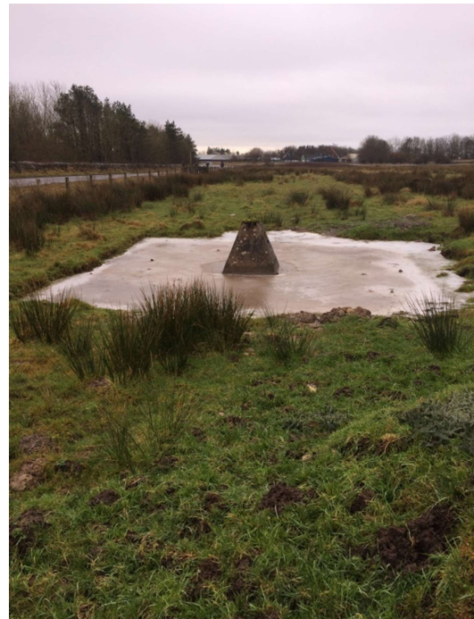
Capped Mine Shaft
