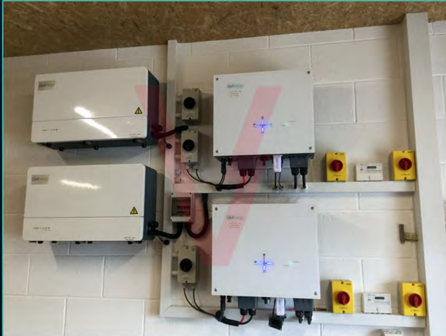
2 x 5kWh Hybrid Inverter 2 x 6.3kWh Battery
