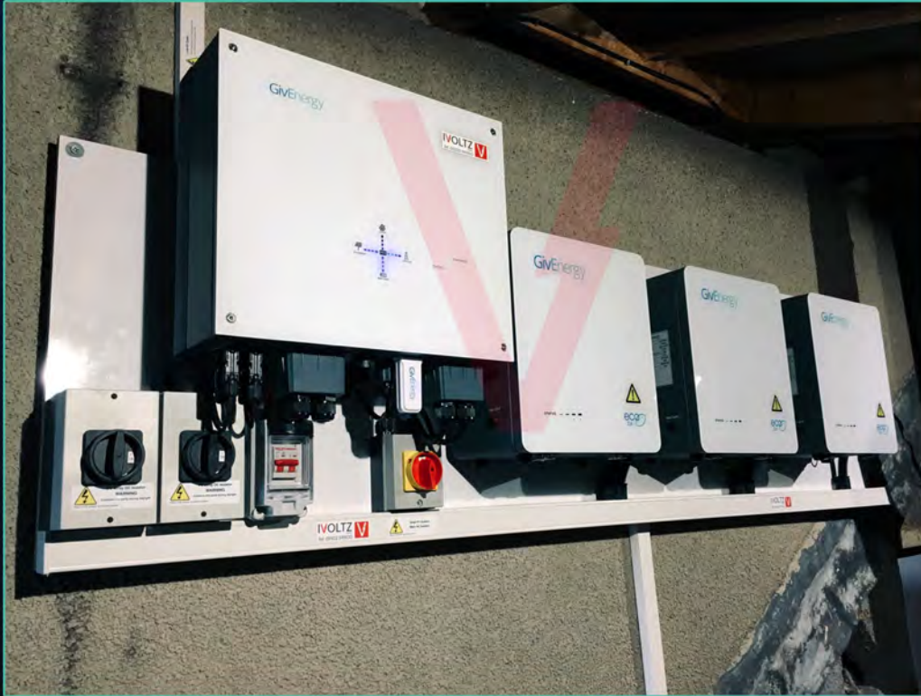
5kWh Hybrid Inverter 3x2.6kWh ECO Battery
