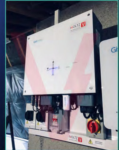
5kWh Hybrid Inverter 3x2.6kWh ECO Battery
