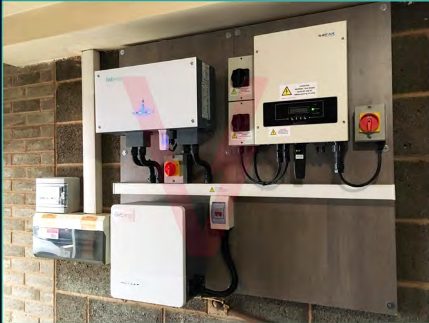
AC Coupled + 2.6kWh Battery
