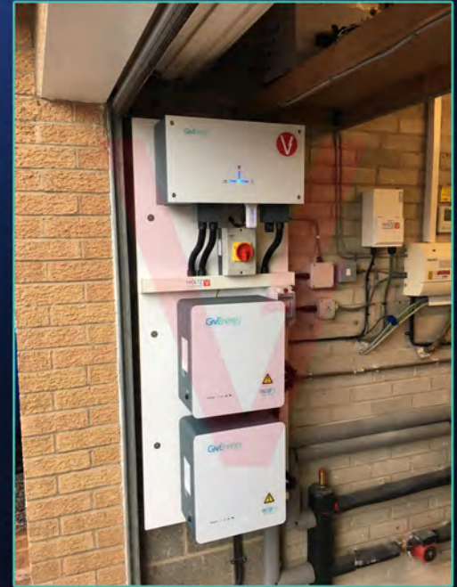
AC Coupled + 2x2.6kWh ECO Battery
