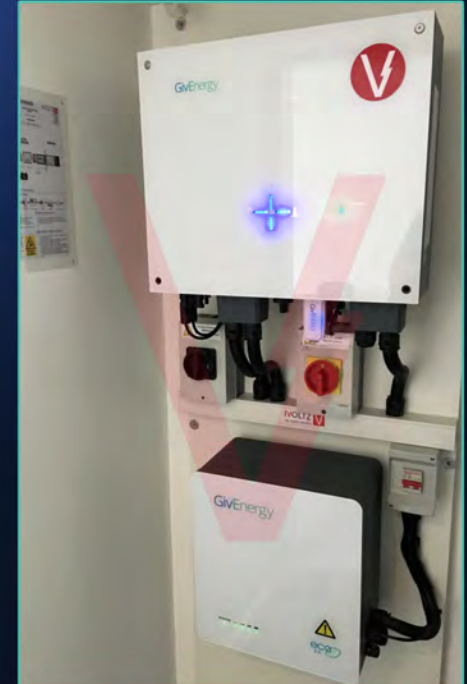
5kWh Hybrid Inverter 2.6kWh ECO Battery
