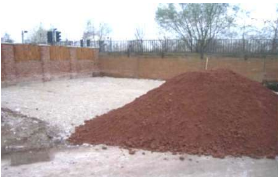
Photograph 10: Inert crushed sandstone being delivered with visible remediation break layer. The spatial area of the remediation can be observed from these photographs (traffic lights).
