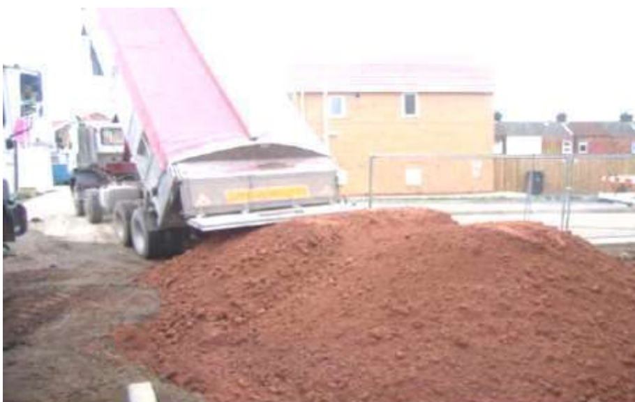
Photograph 9: Inert crushed sandstone being delivered. The spatial area of the remediation can be observed from these photographs (old terrace housing).
