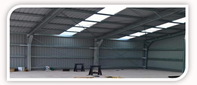
The roof sheets on our single skin buildings are also available with "Dripstop" anticondensation membrane on reverse. Whilst this does not completely eliminate moisture build up the membrane does hold moisture and allows natural venting. The system includes a comprehensive range of fixings, sealants, guttering, flashings and rooflights.
