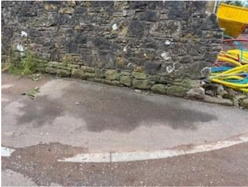
PHOTOGRAPH OF MISSING POINTING AT BASE OF WALL FACING ARLECDON ROAD.
