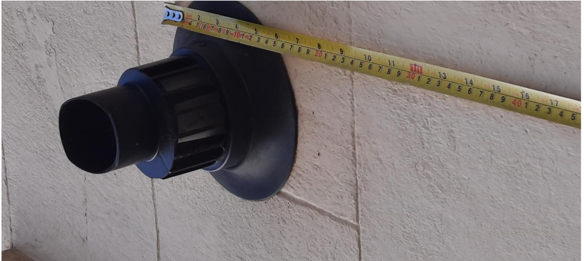
The flue size is approx 7" dia and protrudes from the surface by about 7"
