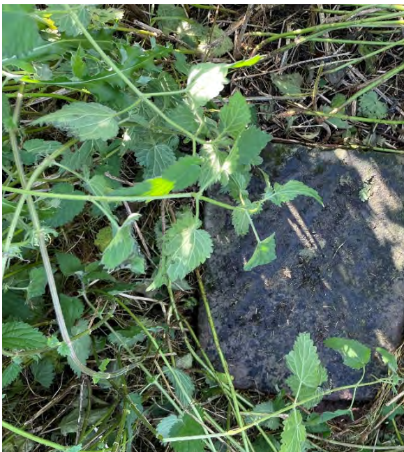
Photo 11: Exiting covered overflow pipe on land drain
