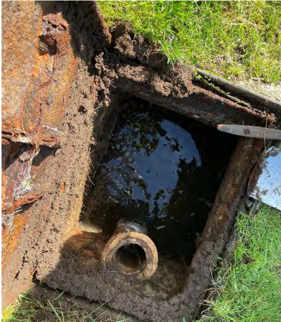
Photo 9: Existing septic tank
