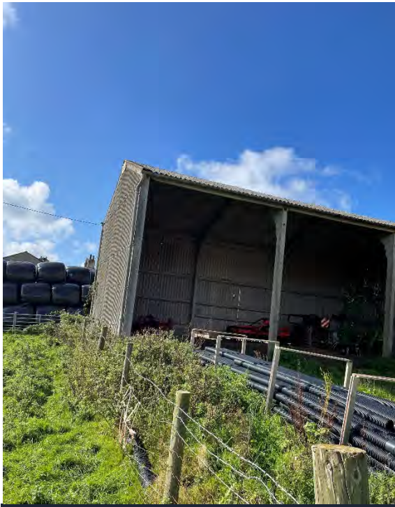
Photo 5: Existing Dutch Barn
