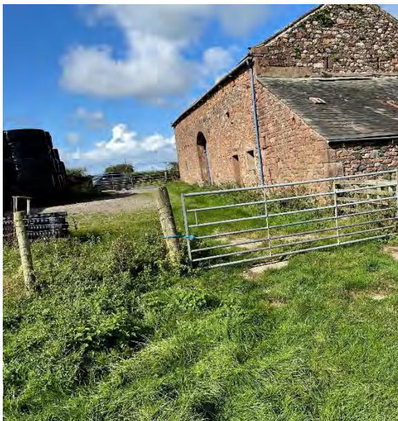
Photo 7: Existing Stone Barn
