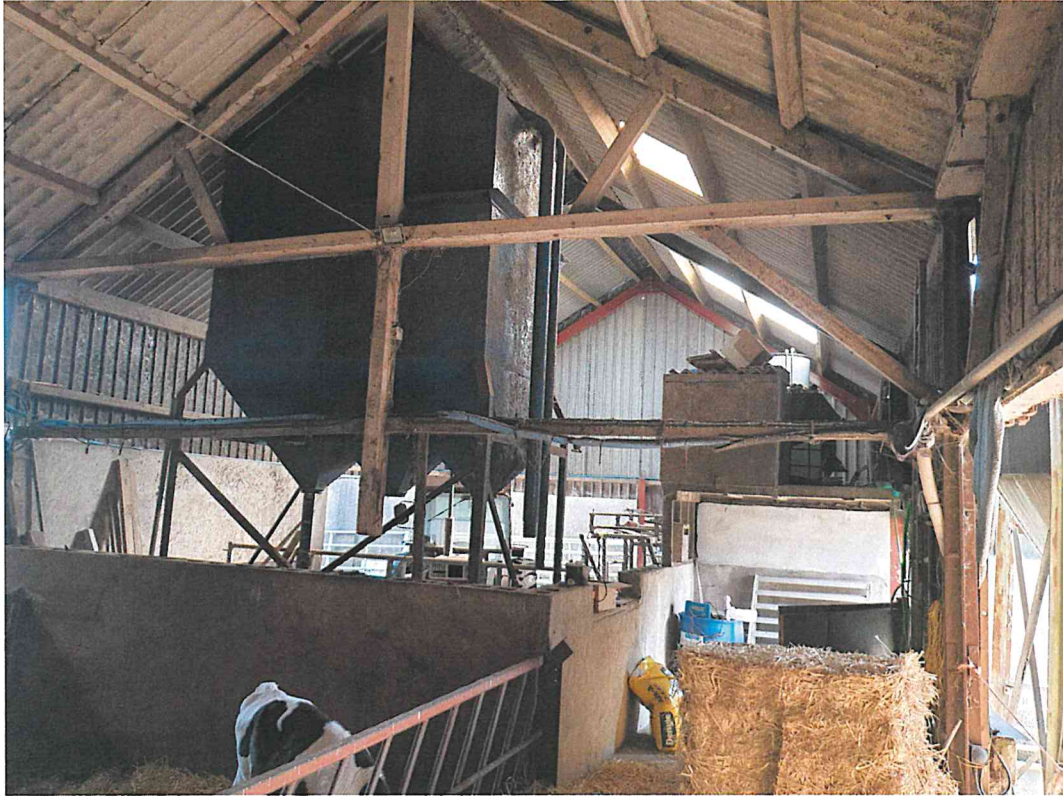
PHOTO 05 VIEW ON THE INCOMPLETE TIMBER GABLE POST
