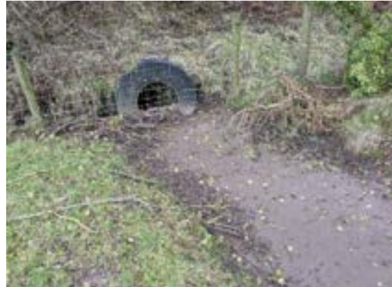
Photograph 8: Culvert under the cycle route embankment (23.02.2025).
