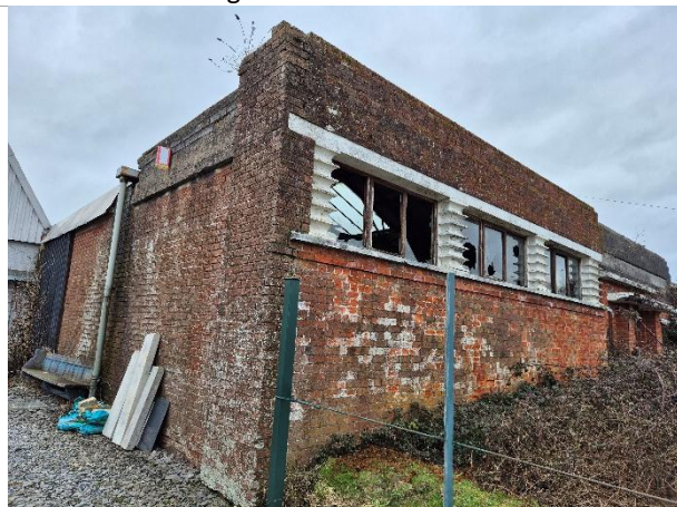
Photo 3: Southern and eastern elevations of the building
