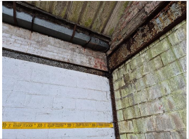
Photo 10: Well pointed internal concrete block walls; no potential roost features
