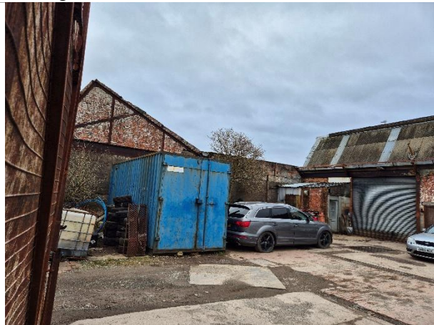
Photo 5: Western elevation of the building
