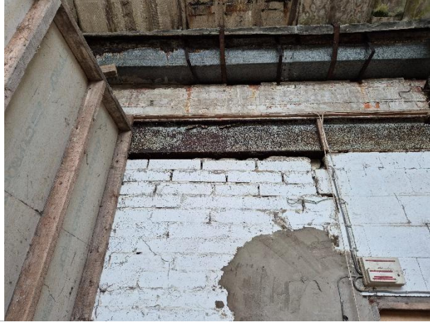
Photo 13: Occasional gaps in internal walls were inspected
