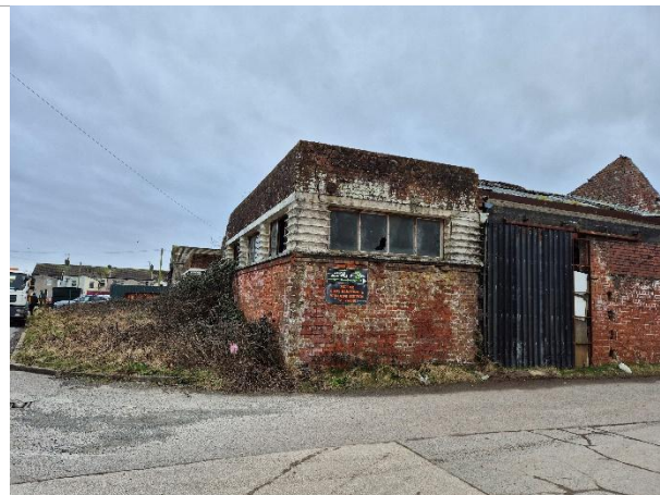
Photo 4: Eastern and northern elevations of the building
