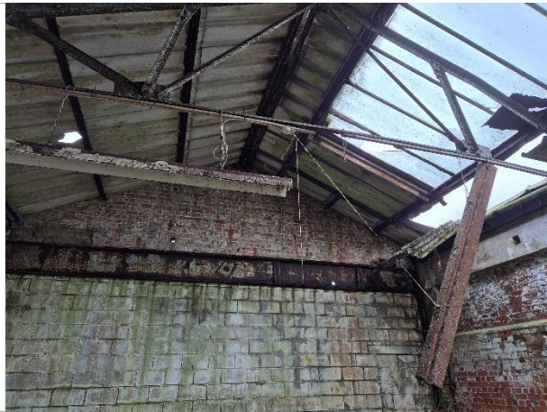
Photo 9: Interior of northern section showing skylights
