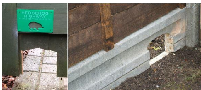
Insert 1: Showing wildlife access gap within fencing
