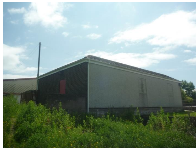
Photo 26: Building 2, north-eastern and north-western elevations
