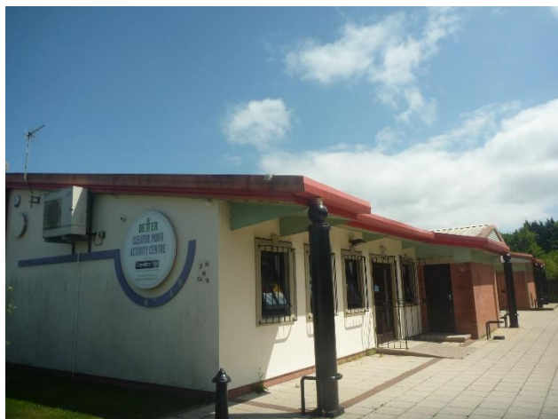
Photo 19: Building 1, south-western (front) elevation
