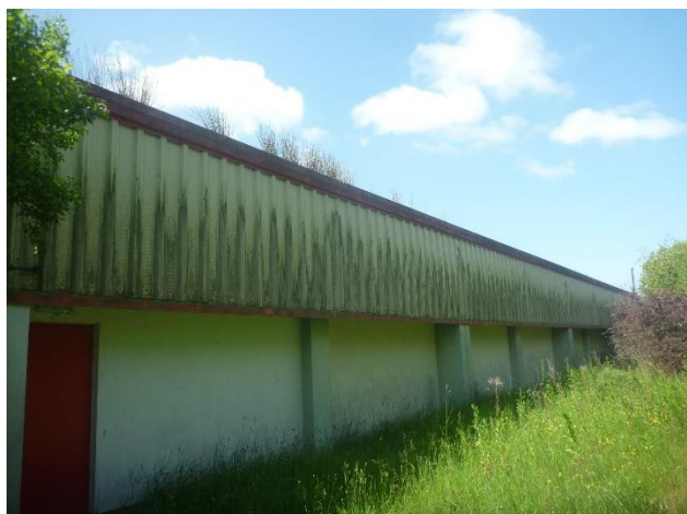
Photo 21: Building 1, north-eastern elevation
