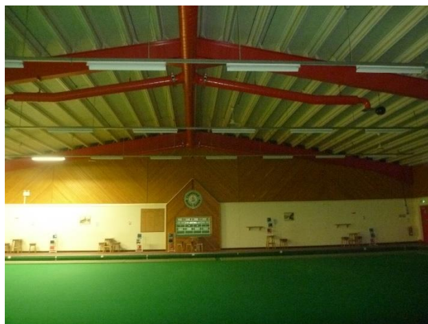
Photo 24: Building 1, internal area, facing south-east
