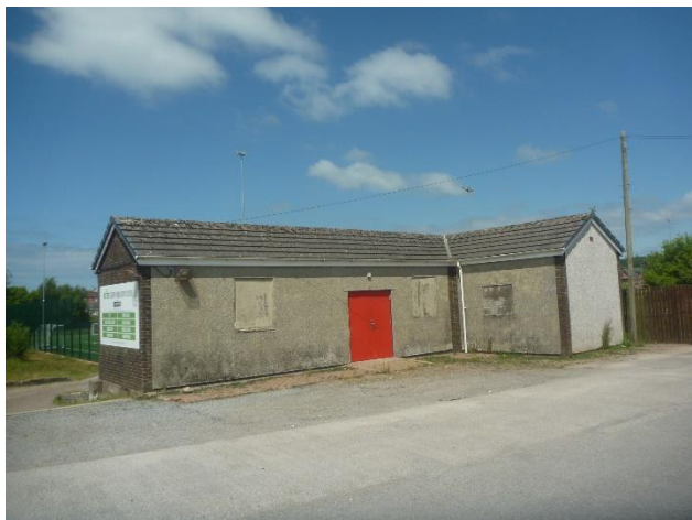
Photo 25: Building 2, south-western and south-eastern elevation
