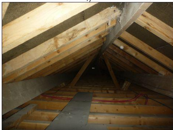
Photo 29: Roof void in Building 2
