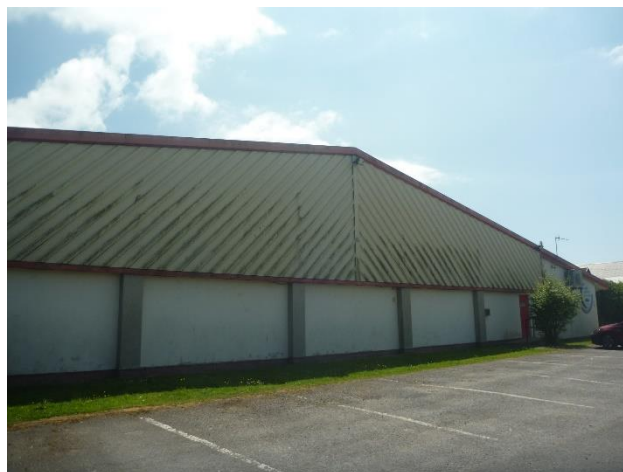
Photo 20: Building 1, north-western elevation
