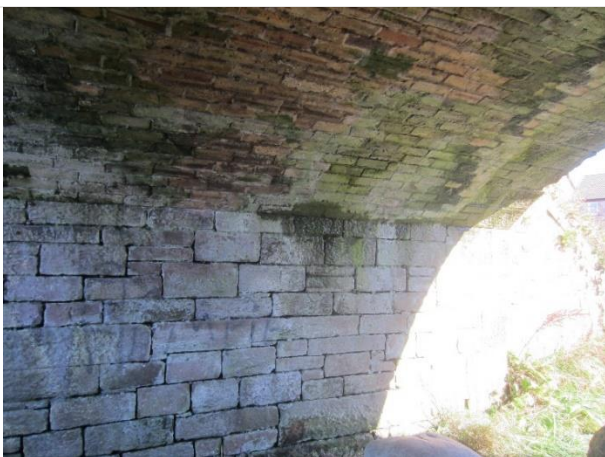
Photo 25: Stone bridge and abutments at the former mineral line (Target Note 9)
